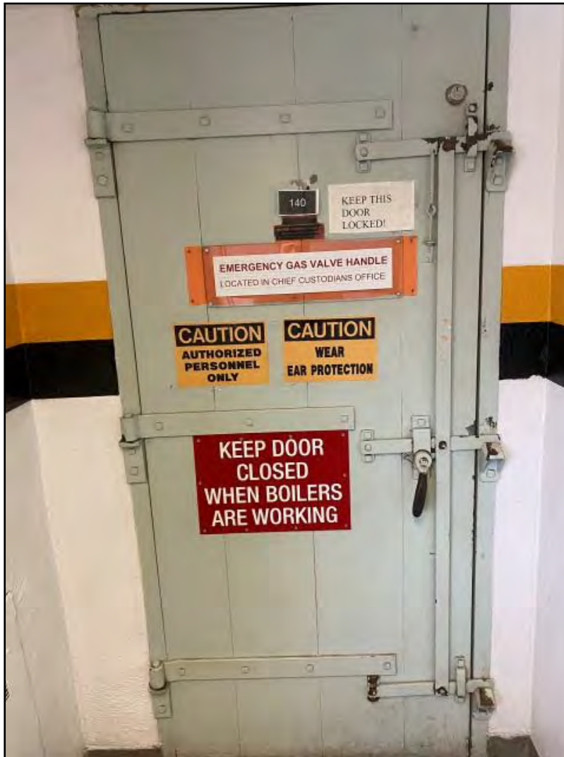
Photograph 7: View of the door to the boiler room.
