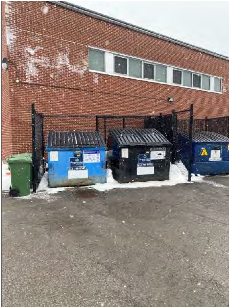
Photograph 24: Looking east at the dumpster storage area on the south side of the school.
