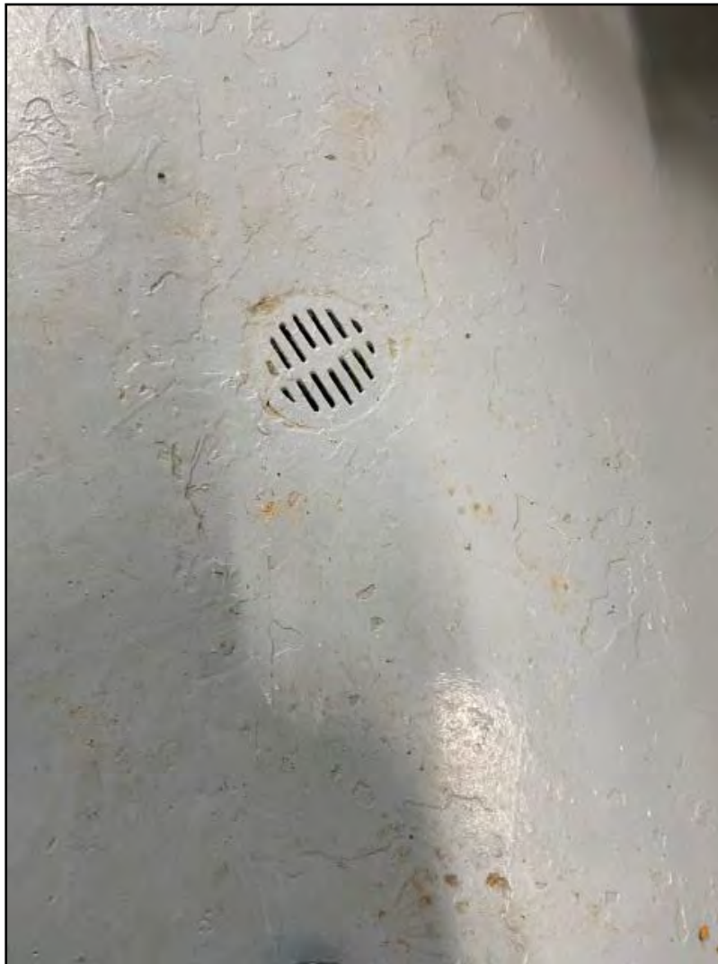
Photograph 12: View another floor drain in the boiler room.
