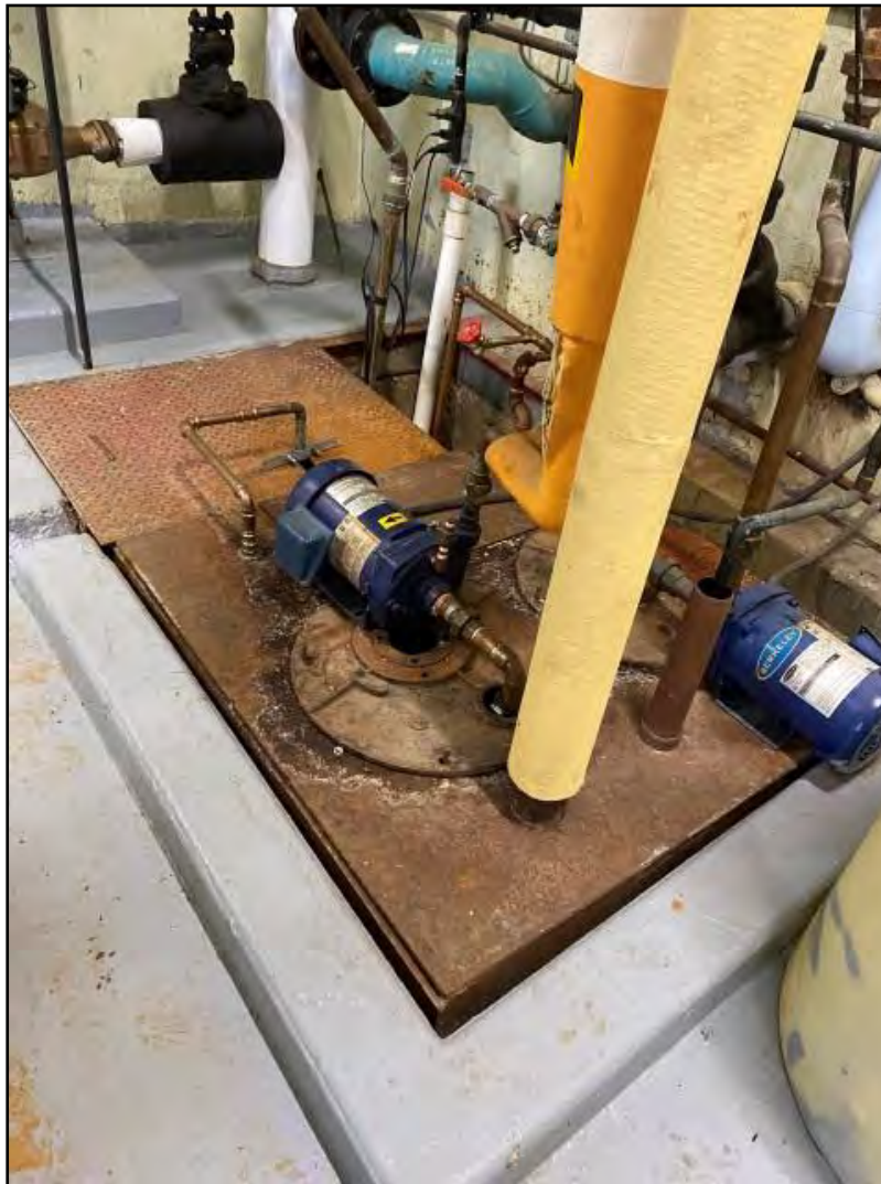
Photograph 10: View of the sump pit in the boiler room.
