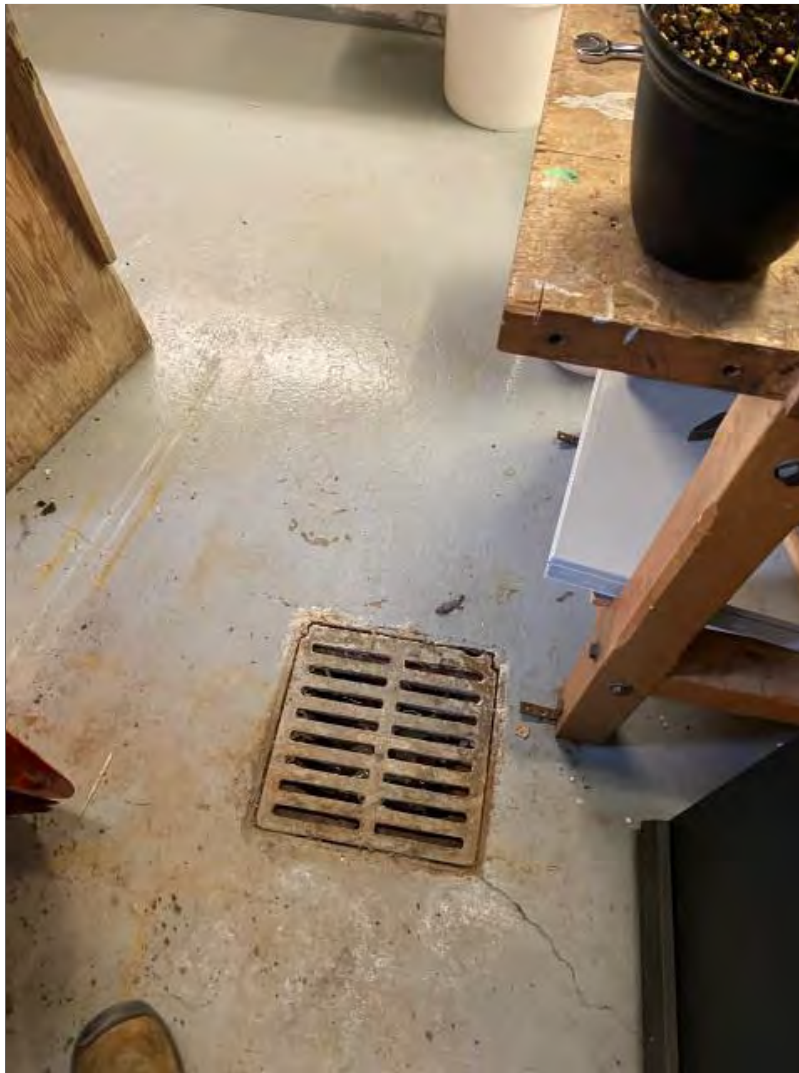
Photograph 19: View of a floor drain in the custodial equipment storage room.
