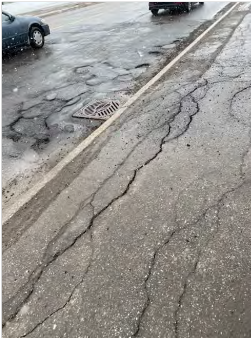
Photograph 28: View of a stormwater catch basin on Smyth Road.
