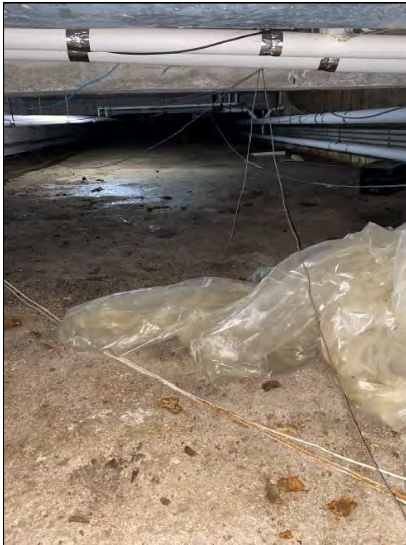
Photograph 16: View of the crawlspace under the building.
