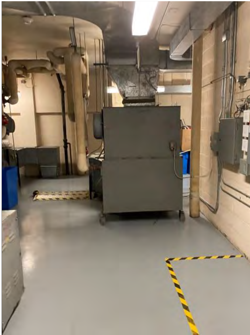
Photograph 18: View of a HVAC/electrical room on the second floor.
