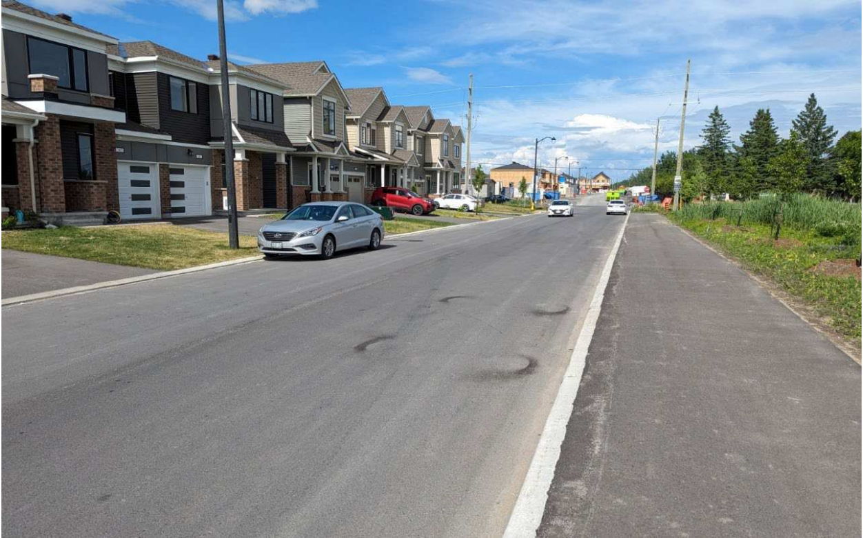
Figure 4: View facing east on Sweetvalley Drive, west of Tenth Line (June 2023)
