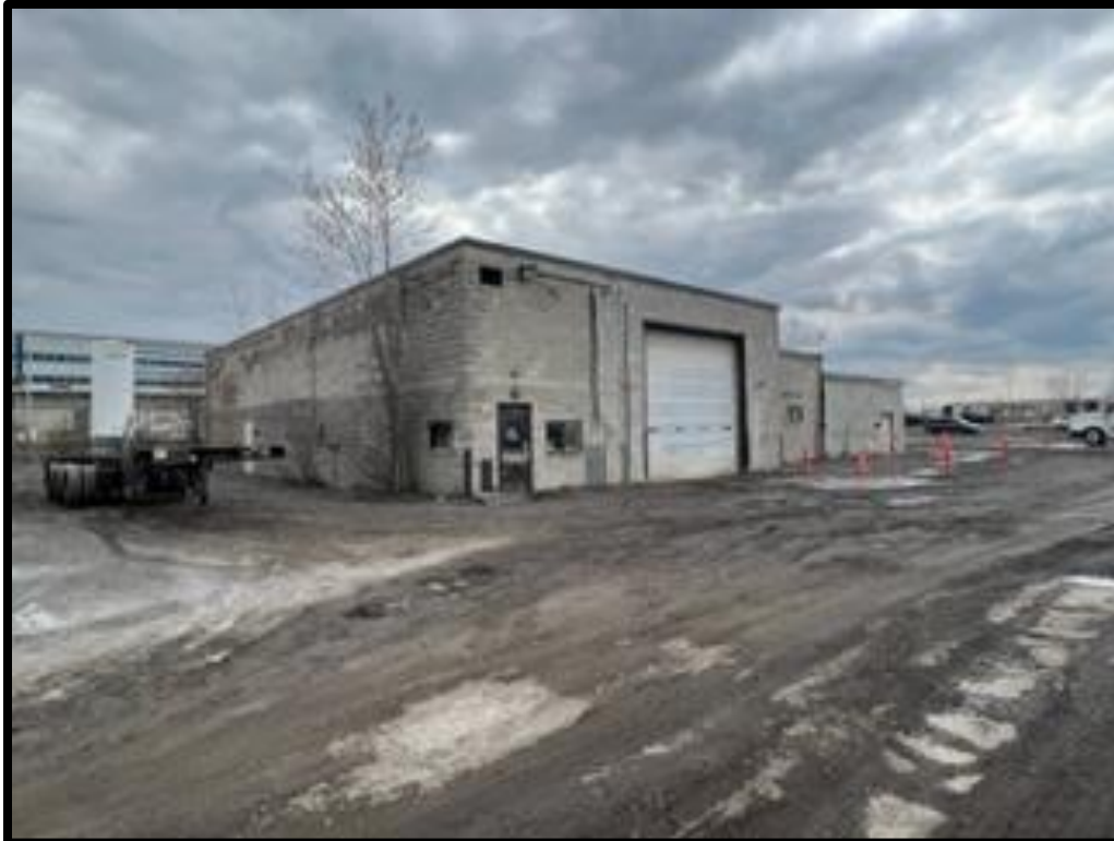
Photograph 2: View of the garage building with maintenance bays on the eastern portion of the Phase I Property.
