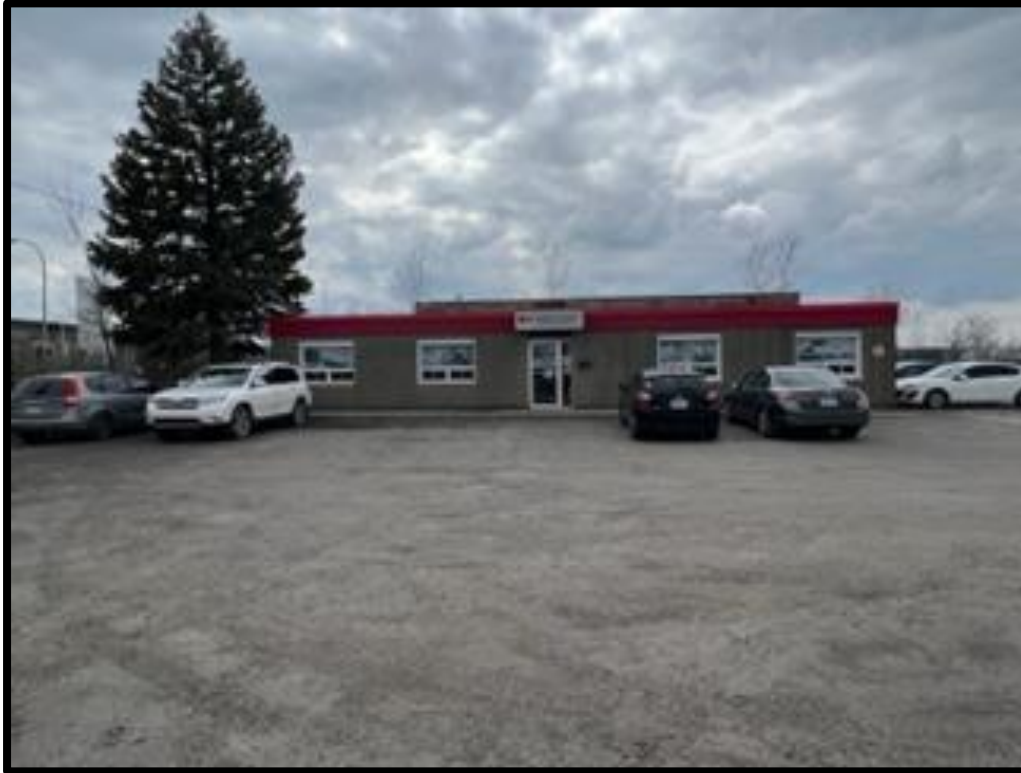
Photograph 1: View of the eastern portion of the Phase I Property, facing west.
