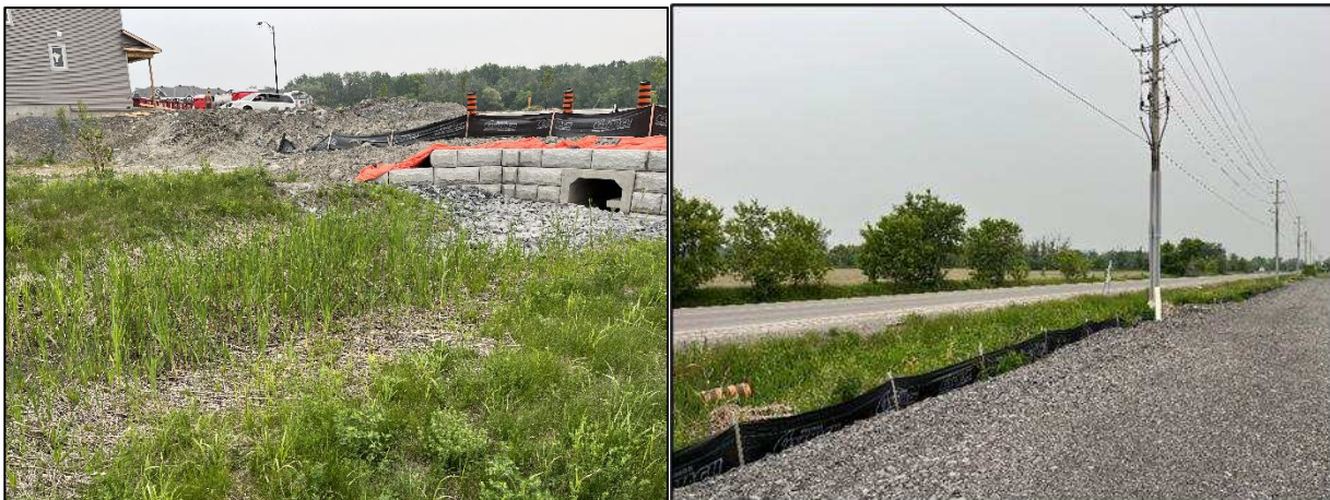
Photos 1 & 2: Photo 1 - East side of Subject Property - Drainage Feature for Jock River on adjacent (east) property (looking southeast). Photo 2 - Drainage Feature for Jock River on adjacent property to the west (looking north).
