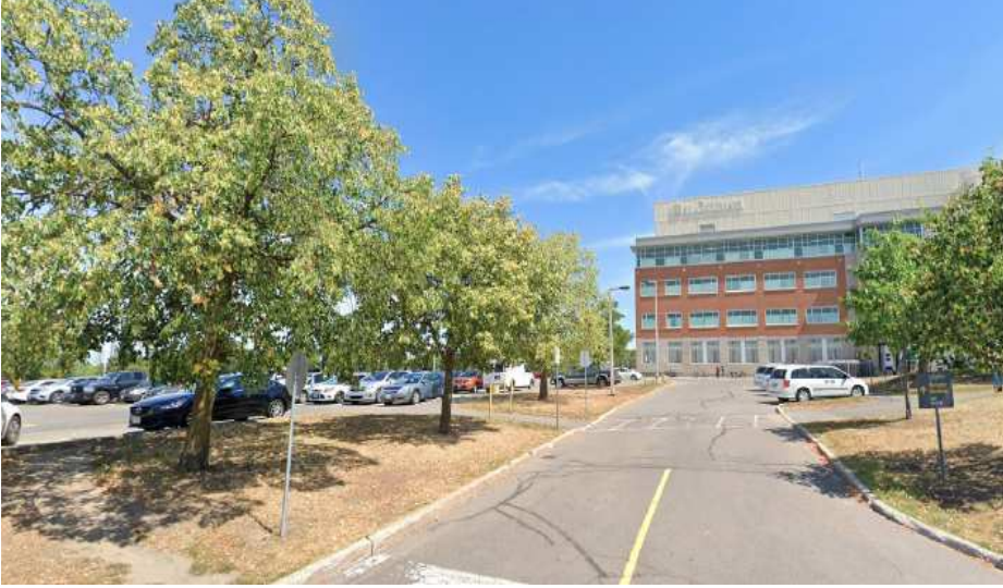
6. View of SW corner of site from access road
