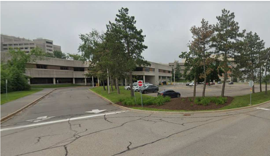
4. View of entrance to Ottawa Hospital Rehab Centre (NE site boundary)
