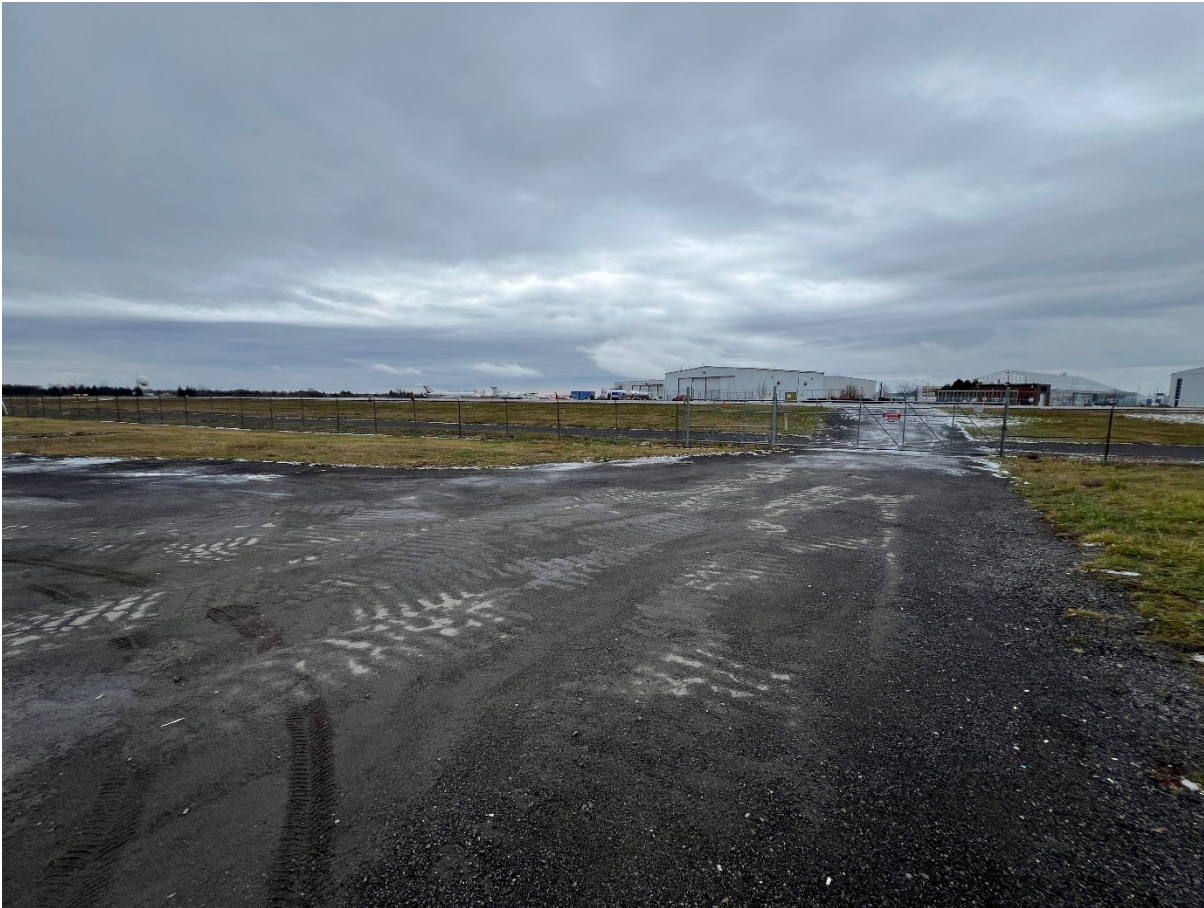
Figure 4 – 02 view looking West toward Taxiway Golf
