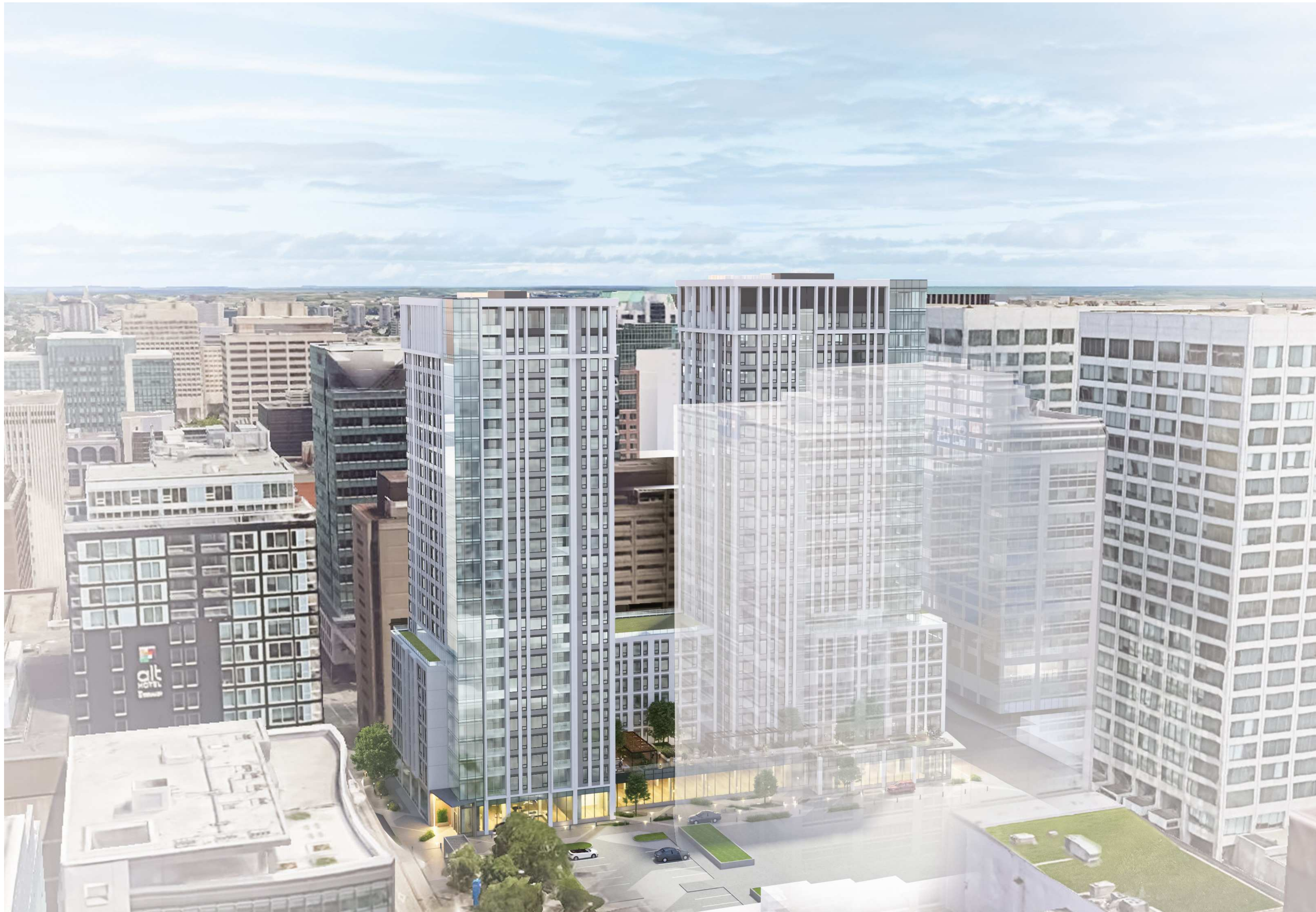
AERIAL VIEW LOOKING EAST
