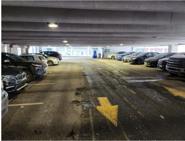
Photo 7 - Inside the garage, ground floor looking north.
