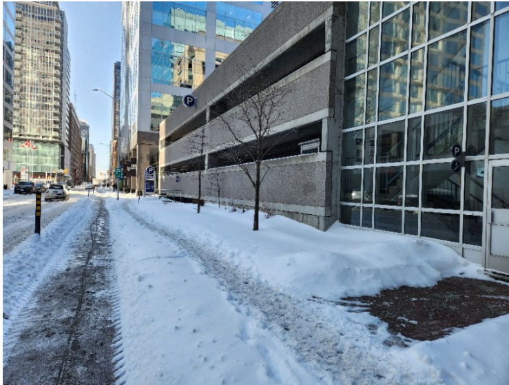
Photo 4 - A view of the south side of the garage, looking west.
