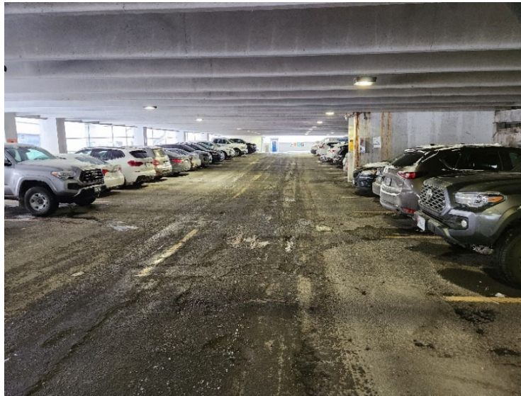
Photo 8 - Inside the garage, ground floor looking south.
