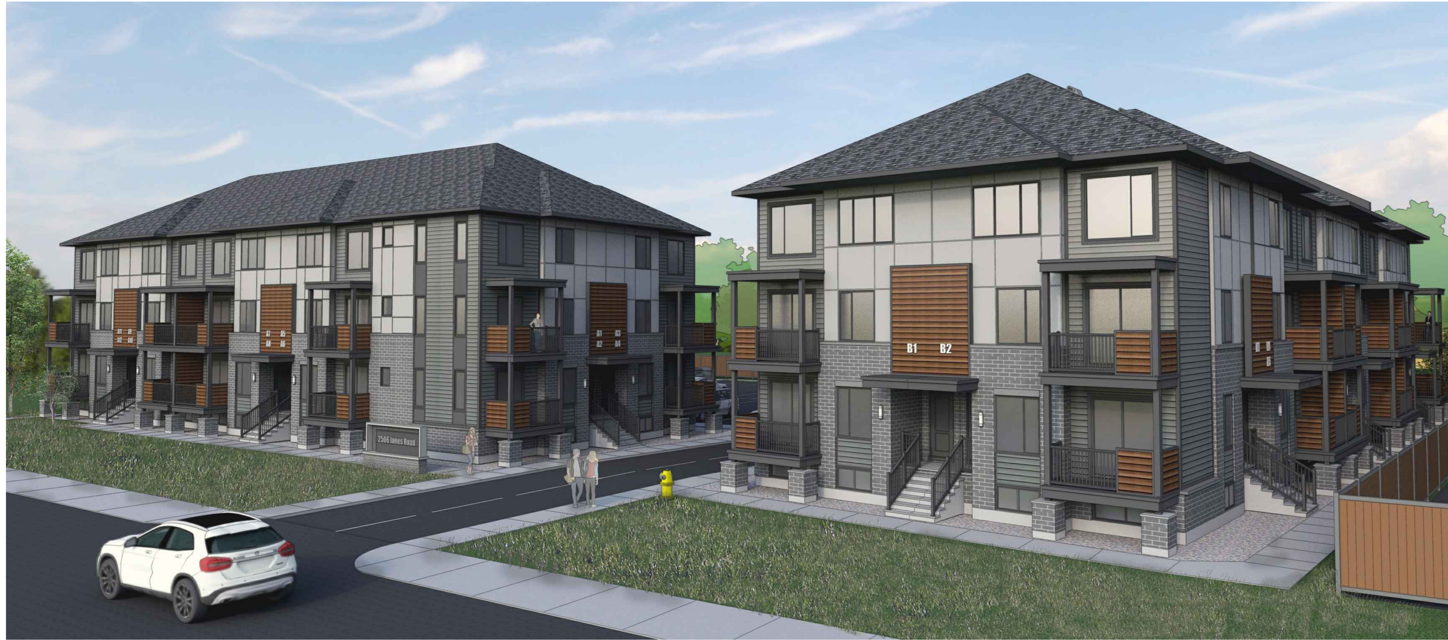
01 | VIEW ALONG INNES ROAD
