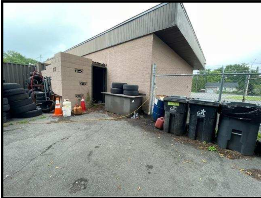
Photograph 7: View of the exterior south wall on the eastern side of the Phase I Property showing the waste oil AST (with 4 tires stacked on top of it).
