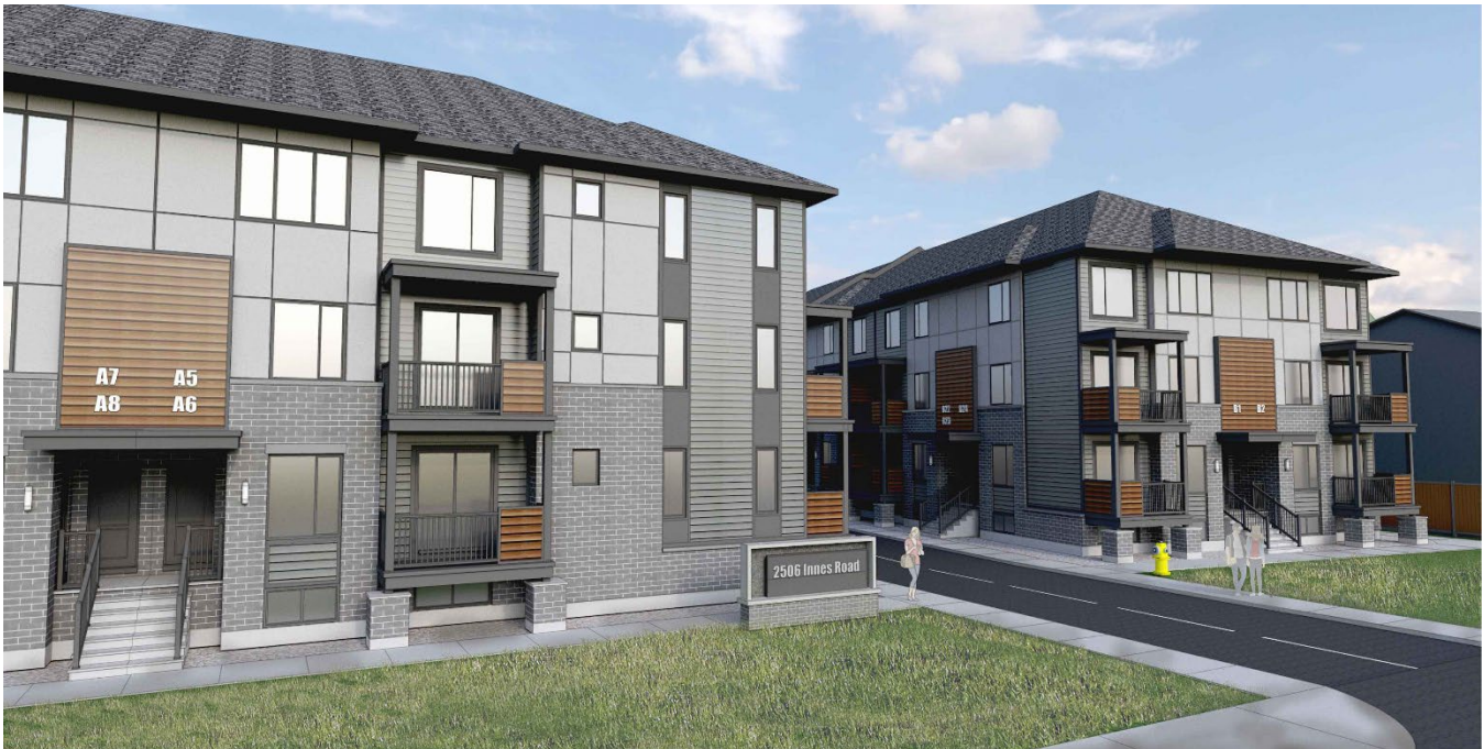
Figure 11: Site Access from Innes Road between Building B and Building A.
