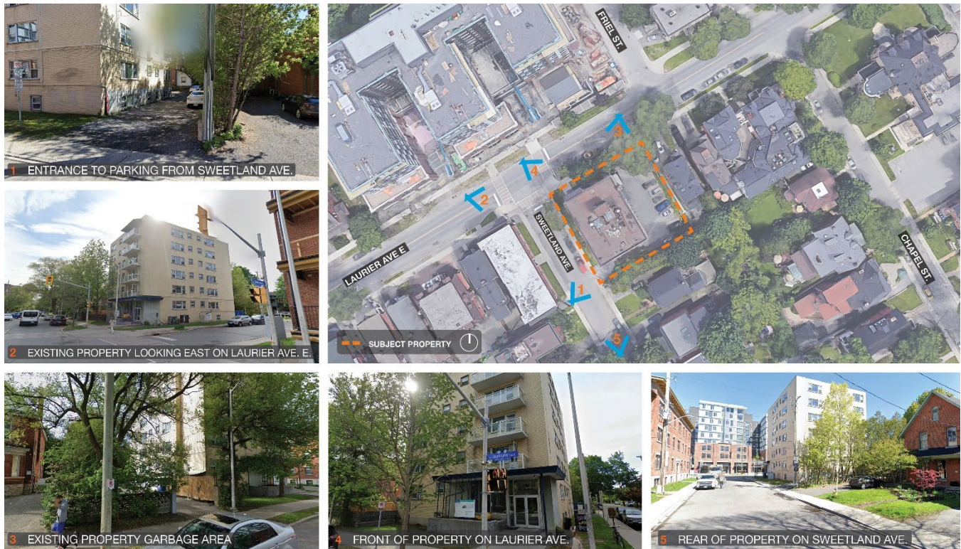
Figure 2: Images of the subject property and surrounding area.
