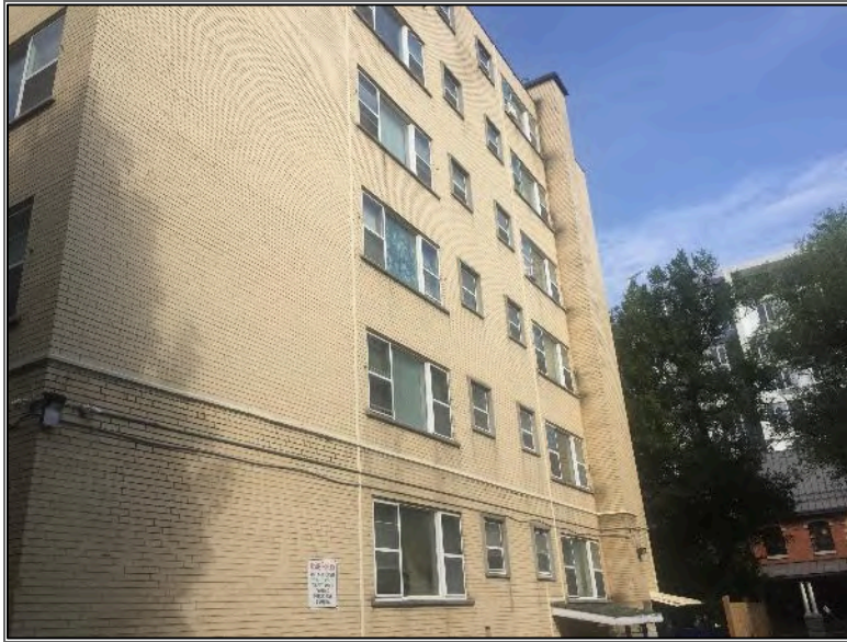
Photo 3 – Site Building (east elevation).
