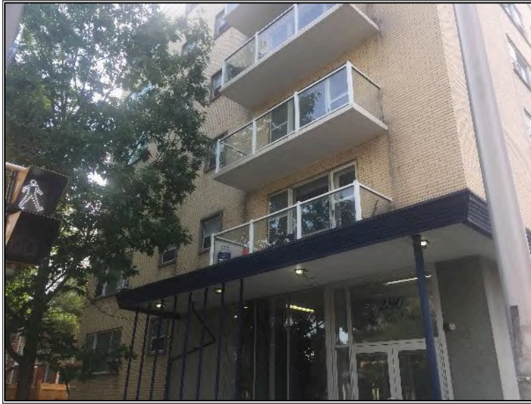
Photo 1 – Site Building (north elevation).
