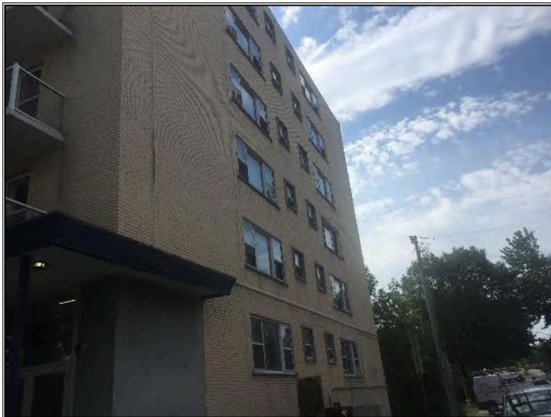
Photo 4 – Site Building (west elevation).
