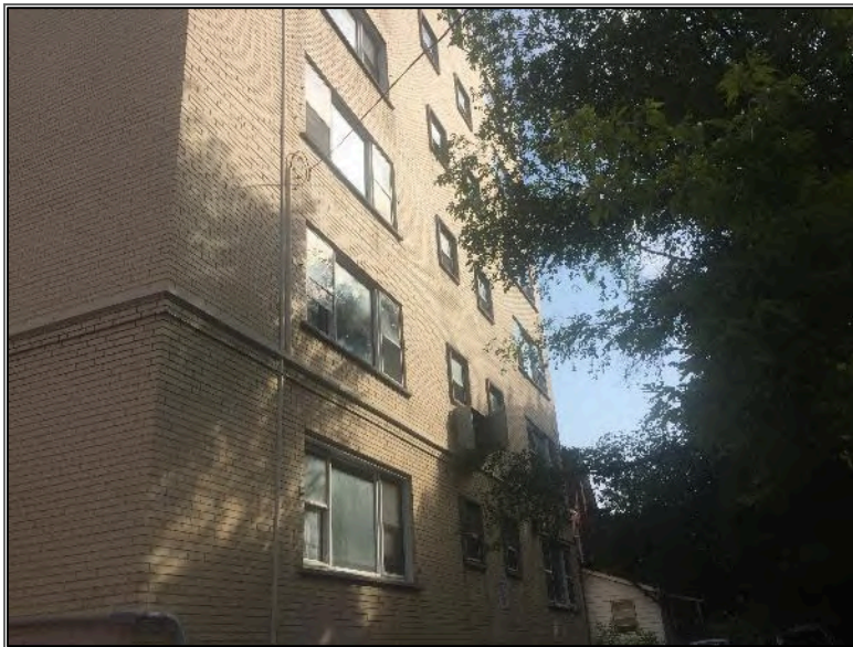
Photo 2 – Site Building (south elevation).
