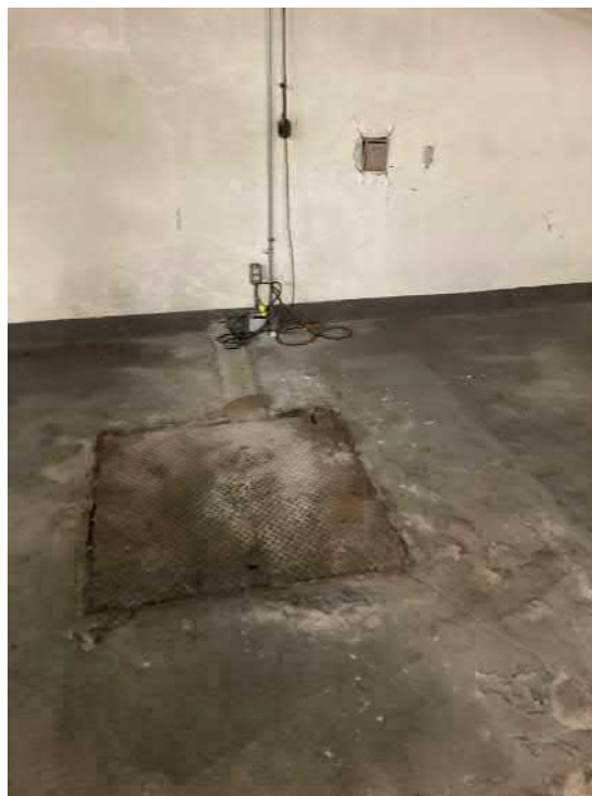
Photo 14: Sump pit in underground parking garage
