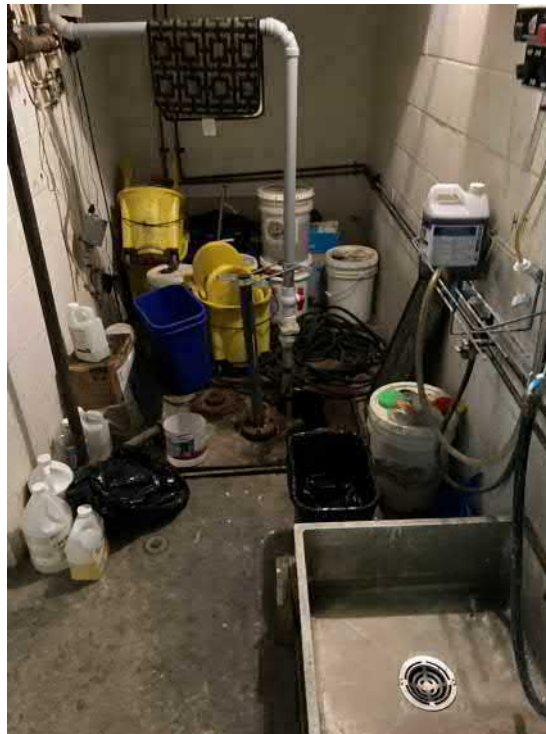
Photo 5: Custodial room basement level, original portion of building, showing sump pit (1 of 2) and commercially-available cleaning products
