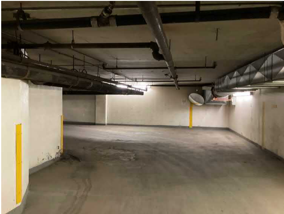
Photo 13: Ramp of underground parking garage, north wall
