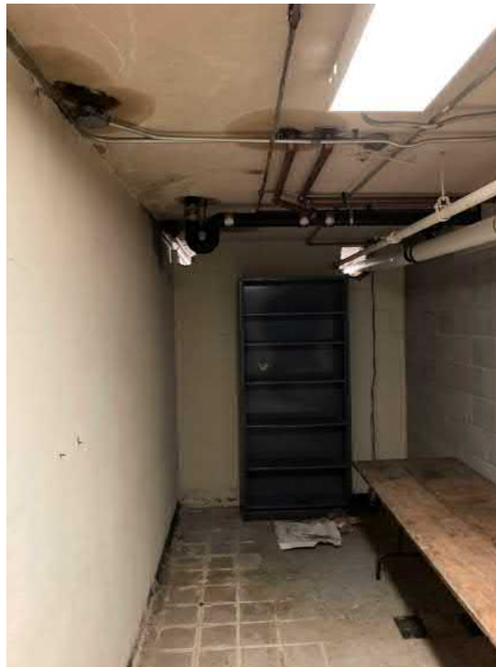
Photo 3: Basement storage room along north building wall, facing east
