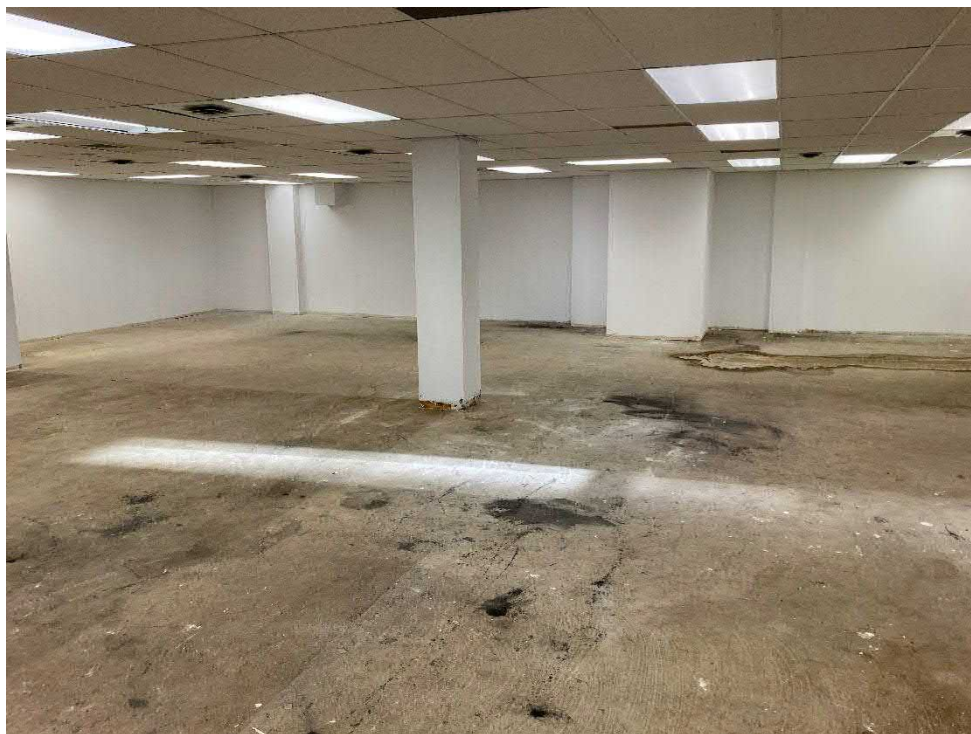
Photo 17: Interior of office unit, undergoing renovation
