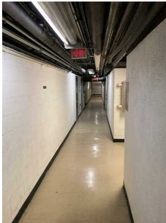
Photo 2: Typical interior of basement level (original portion of building), facing west
