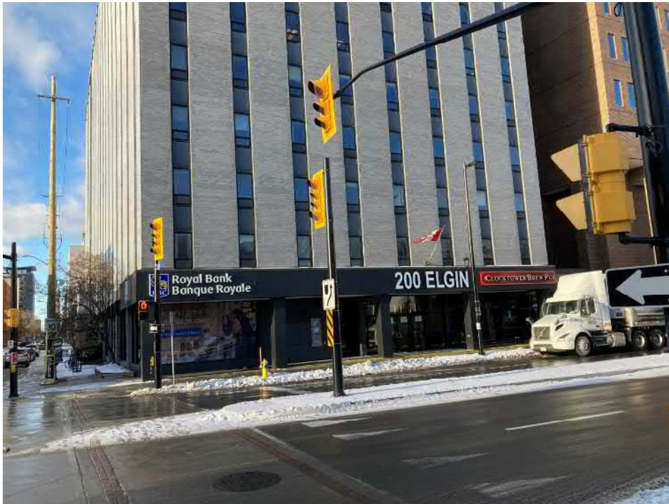
Photo 1: Site building, facing west from Elgin Street
