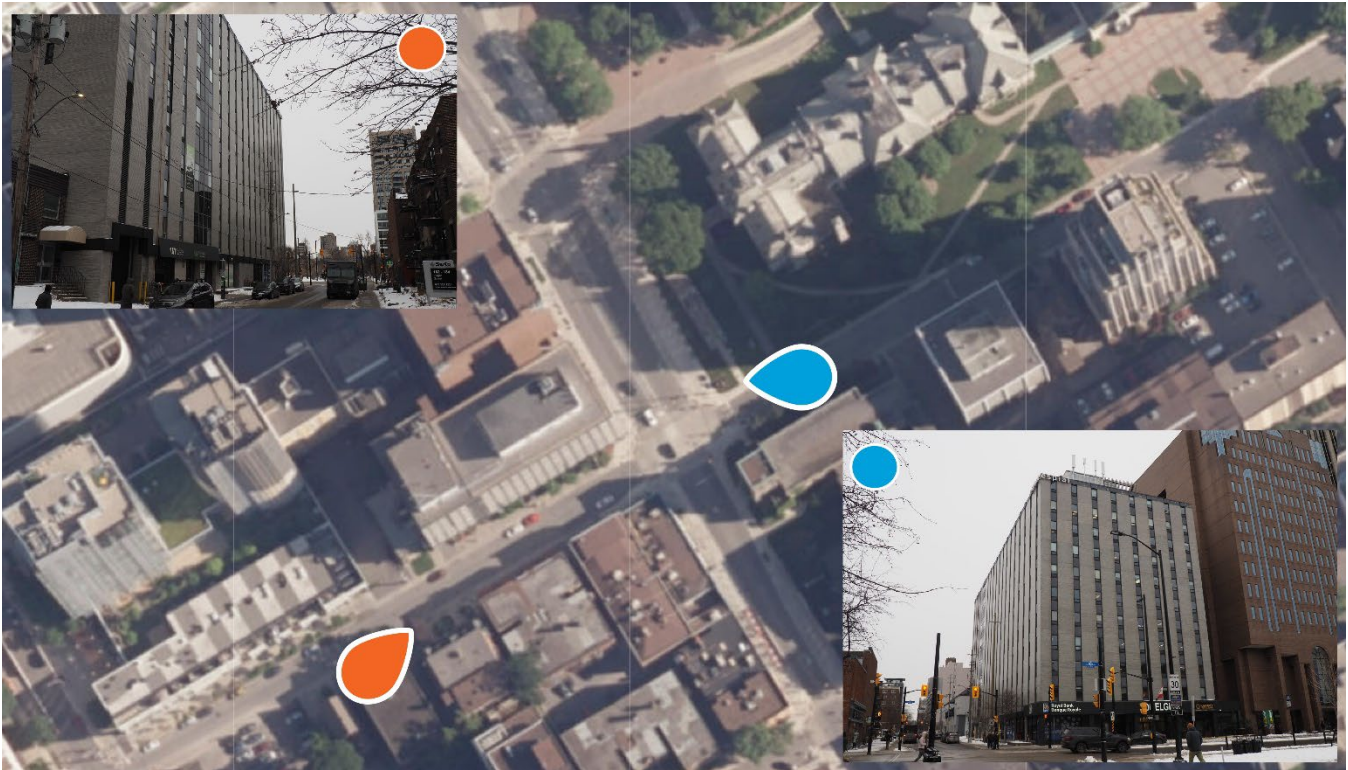
Figure 7: Photos of the Lisgar Street (top) and Elgin Street (bottom) facades of the existing building on the subject property.
