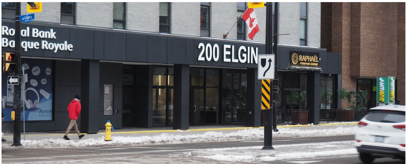
Figure 11: Existing ground floor condition of 200 Elgin Street.
