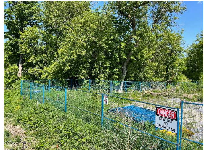
Looking at the northeast corner of the site from the access road along Klondike Road
