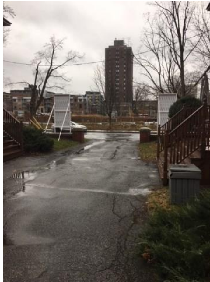
Photo 1: View south from lane in between 283 (left) and 285 (right) McLeod Street. (2020 Site Visit)
