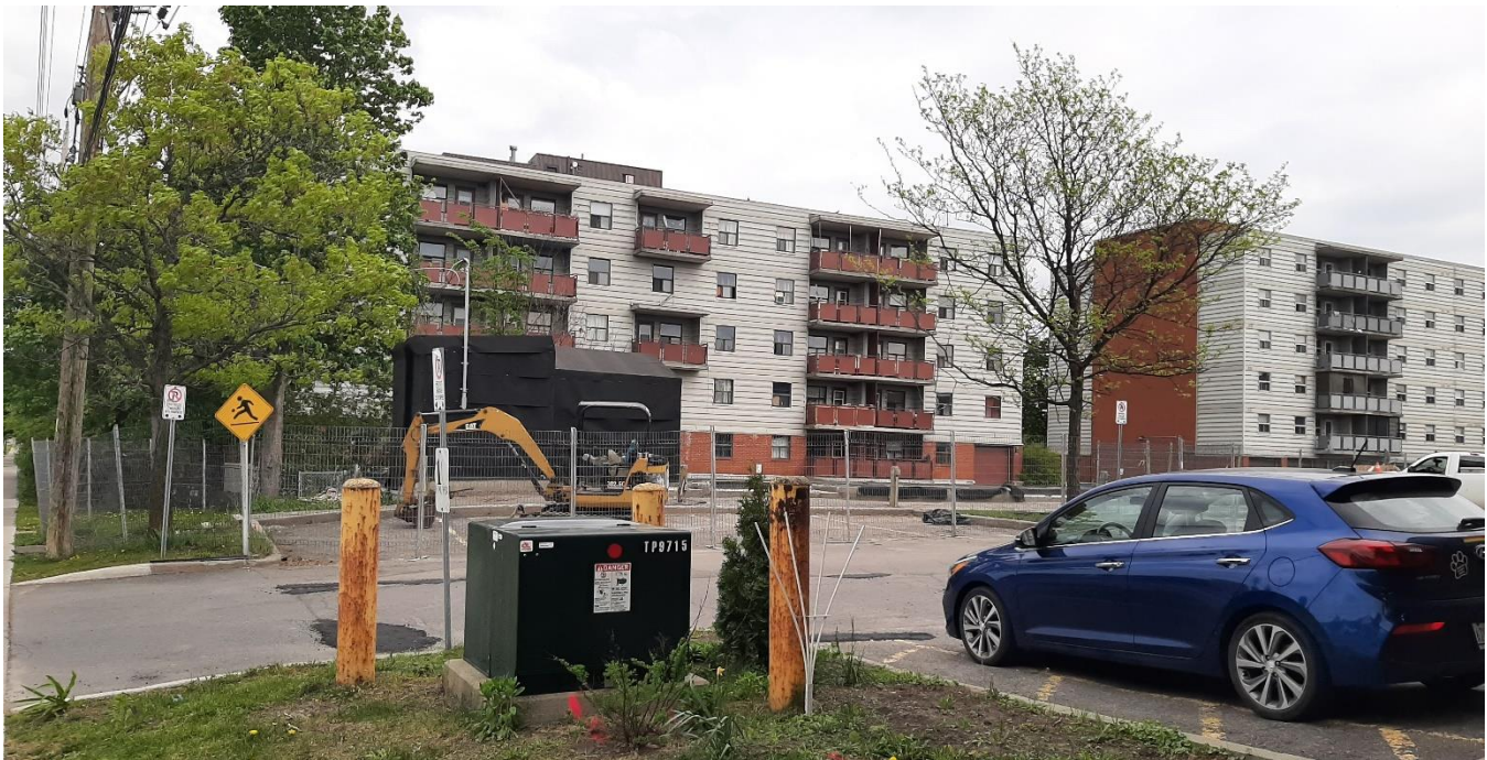
Figure 3: Subject site, with demolished Block 3 in the midground
