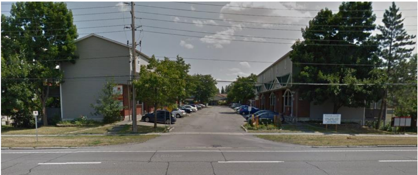
Figure 16: Previous Condition (Google Streetview, July 2018)
