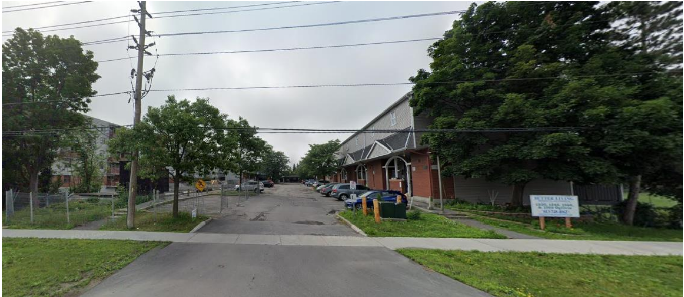
Figure 2: Entrance to the Better Living site, with the two (2) pathways visible, one (1) of which has been fenced off due to the fire; note the staircases leading to the pathways to the right and left of the drive aisle.
