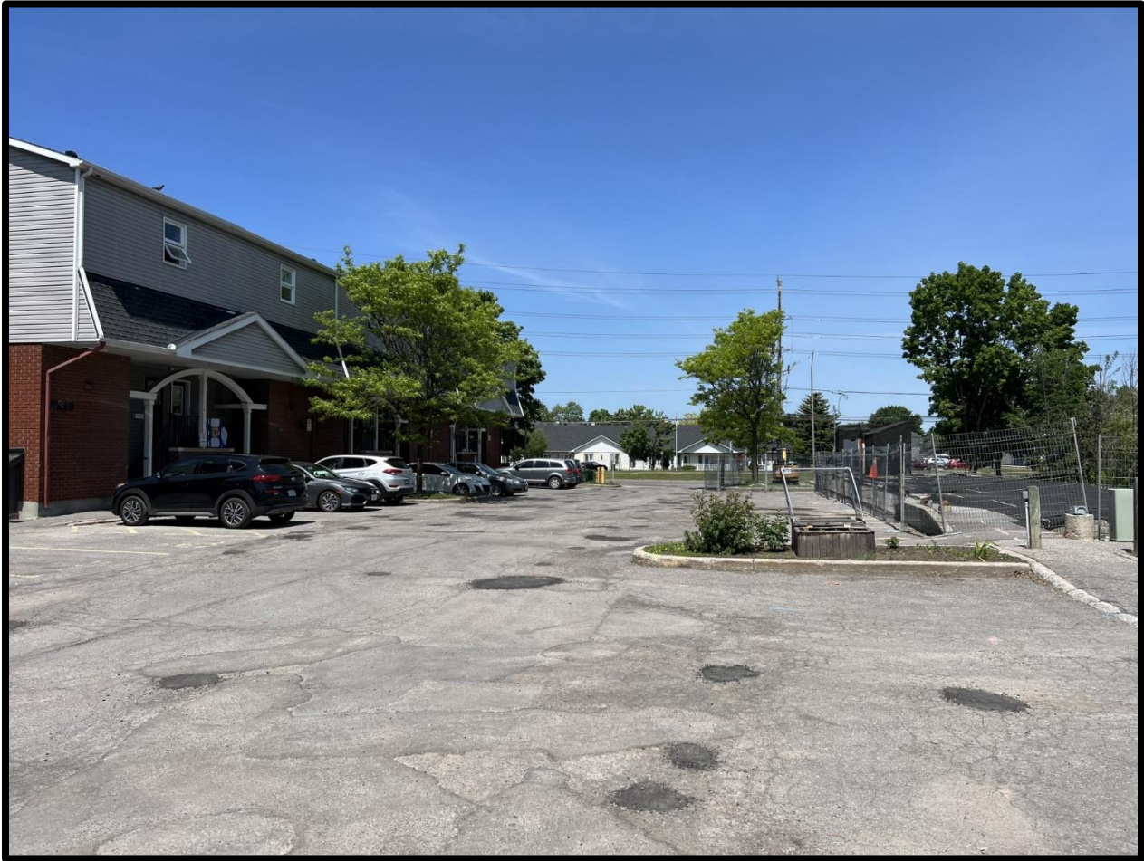
Photograph 1: View of the northern portion of the Phase I Property, facing north.
