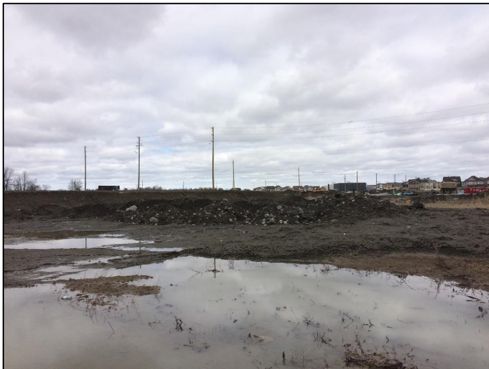
Photo 2: Standing water in east portion of Half Moon Bay West in April 2017.
