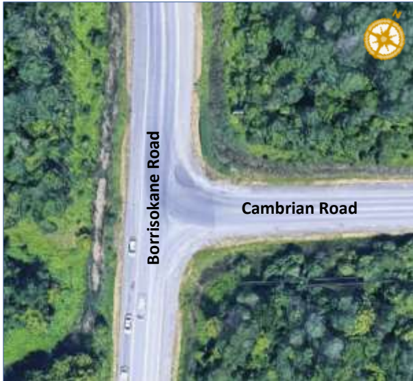
Exhibit 2-4: Borrissokane Road and Cambrian Road Intersection
