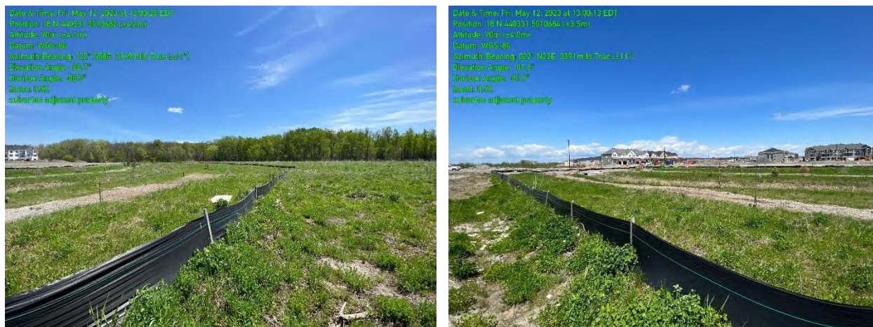
Figure 2 Sediment fencing separating Tipperary Creek (the realigned watercourse) and the Site
