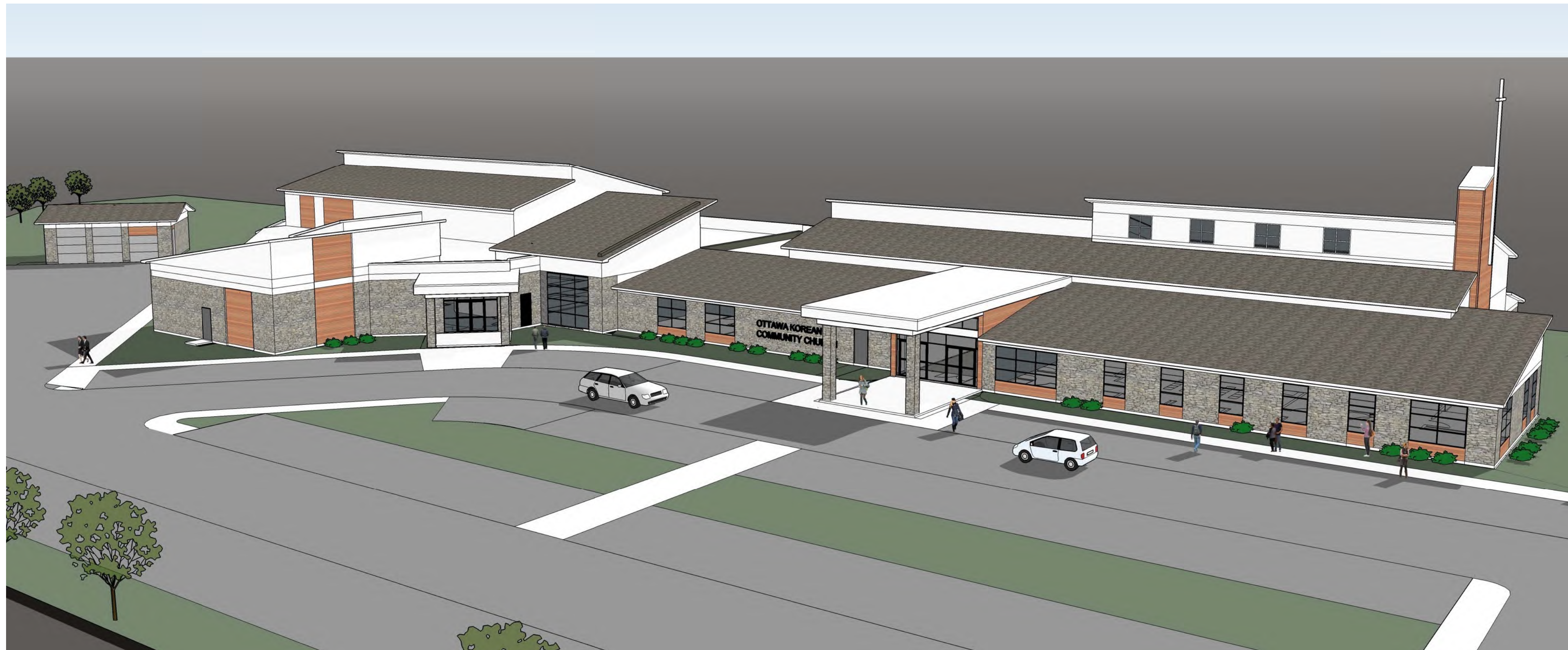
AERIAL VIEW OF NORTHEAST FACADE
