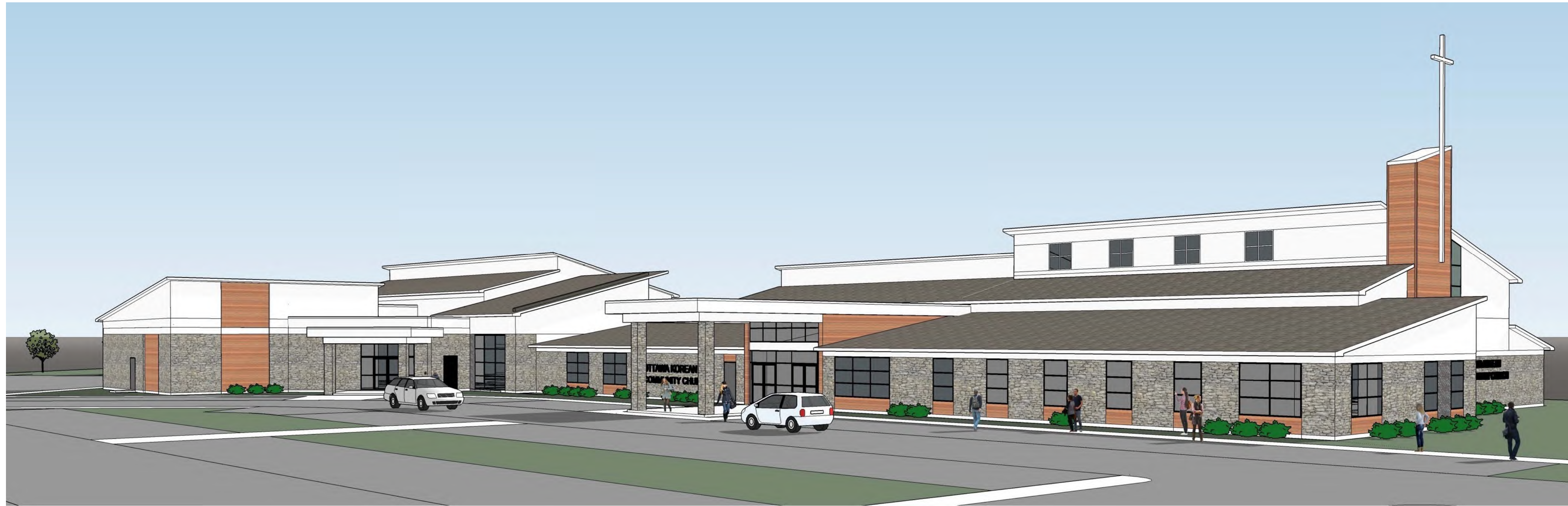
VIEW OF SOUTHWEST FACADE FROM BORRISOKANE ROAD
