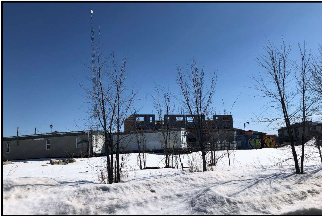
Photograph 4: View of the eastern portion of the 617 Longfields Drive parcel, facing west.
