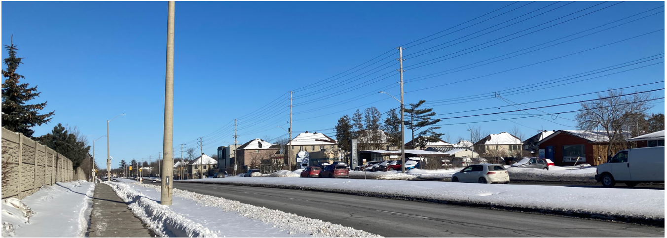
Figure 17: View of Hunt Club Road looking east, with noise wall on north side of the right-of-way visible at left
