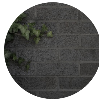
Brick cladding such as "Black Diamond Velour" of Belden or equivalent, "Norman" dimensions.
