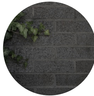
M2 Brick cladding such as "Black Diamond Velour" of Belden or equivalent, "Norman" dimensions.
