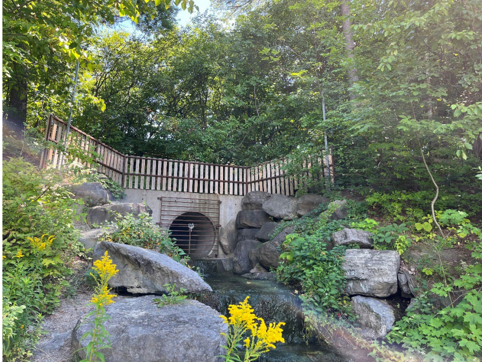
Photo 3. Culvert outlet with discharge onto bedrock at an approximate elevation of 80 m (see Figure 02). Photo taken by BGC 2022-08-15.
