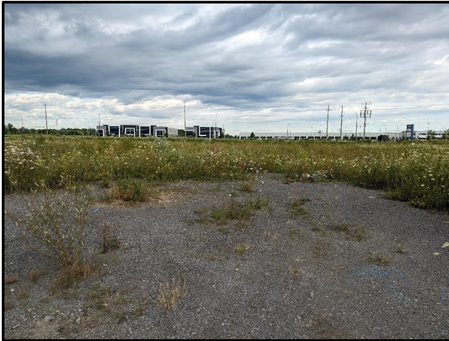
Photograph 3: View of the southern portion of the Phase I Property, facing north.
