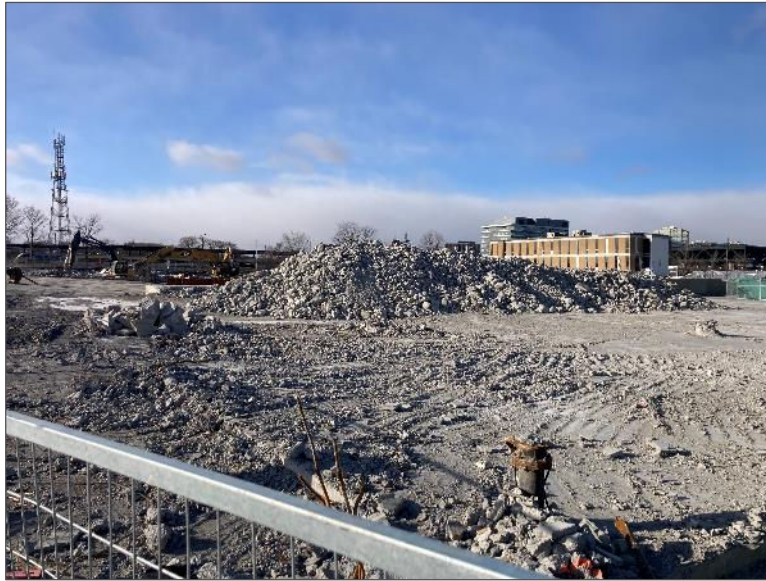
Photo 1 – Building debris/rubble from former Site Buildings (currently being demolished).
