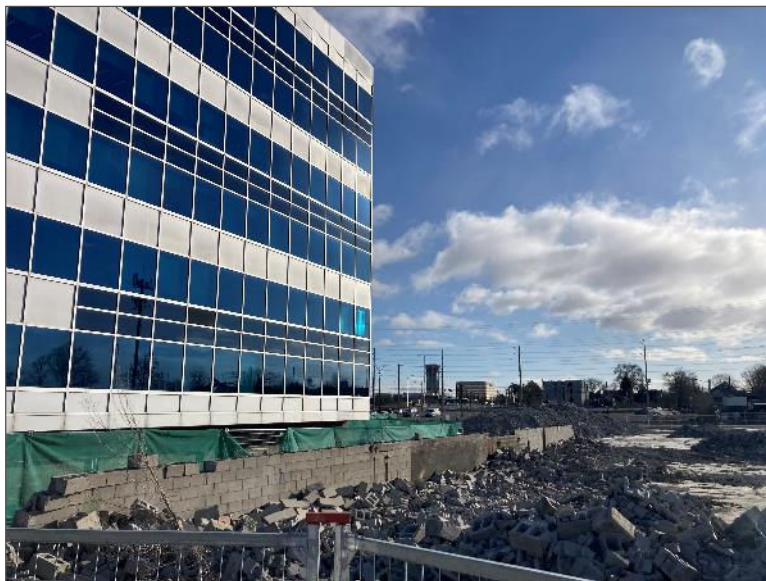
Photo 2 – North adjacent property, looking northeast.
