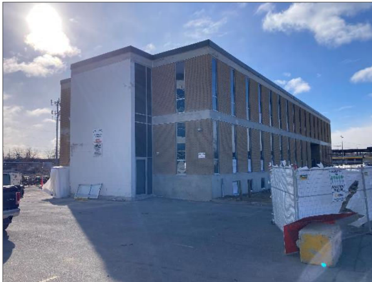
Photo 4 – Site Building C, the only Site Building that currently remains on-Site.
