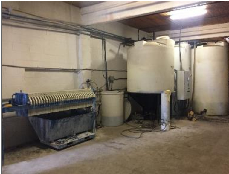
Photo 8 – Three ASTs located within Site Building B that treat the wastewater collected in the trench system/holding tank prior to discharge to the municipal sewer system.
