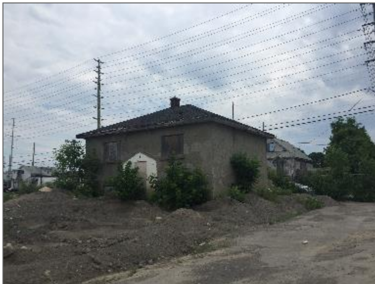
Photo 6 – Site Building F (west elevation).
