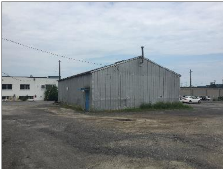
Photo 4 – General view of Site Building D.
