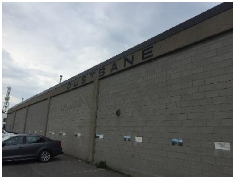
Photo 2 – Site Building B (east elevation).
