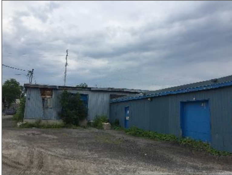
Photo 5 – Site Building E (north elevation).
