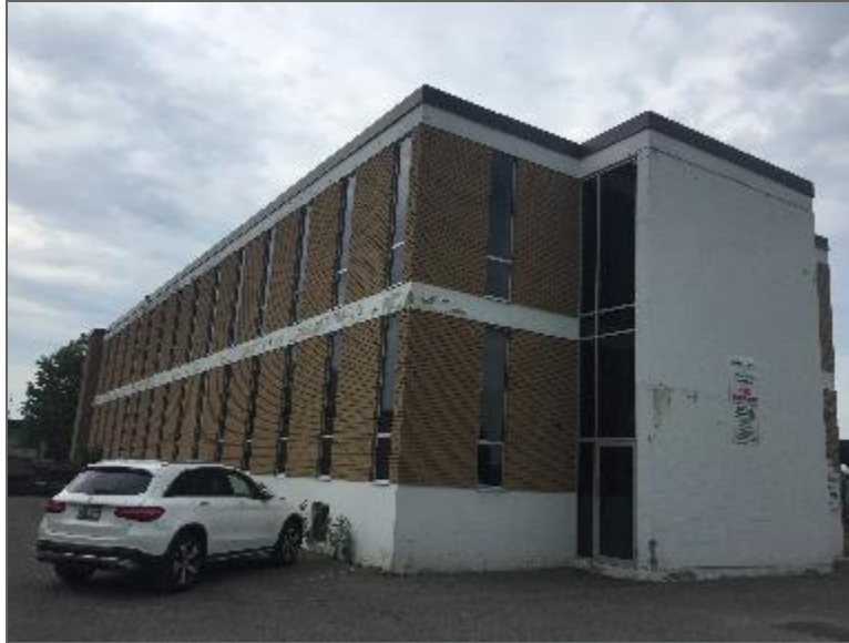
Photo 3 – Site Building C (north and east elevations).
