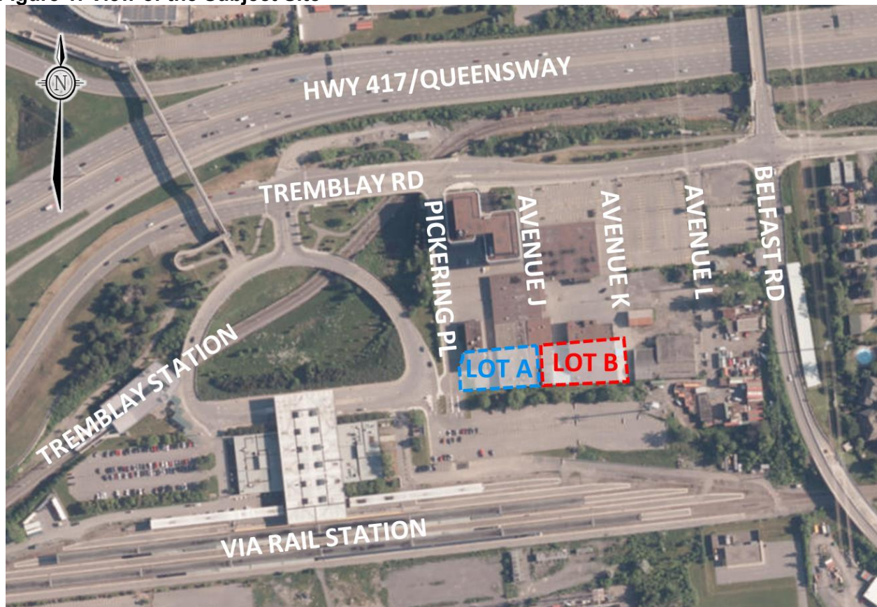
Figure 1: View of the Subject Site
