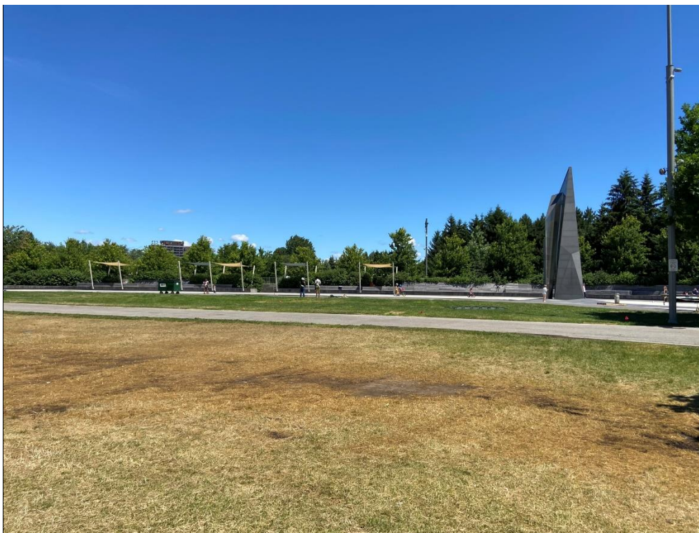
Photo 14: North of Site: General view of the Water Plaza. Date: 06/28/24 Direction: Northeast
