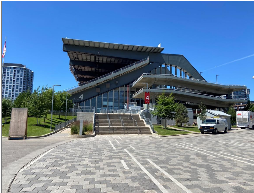
Photo 3: General view of the Eastern elevation of TD Place Stadium and Communications Buildings. Date: 06/28/24 Direction: Southwest
