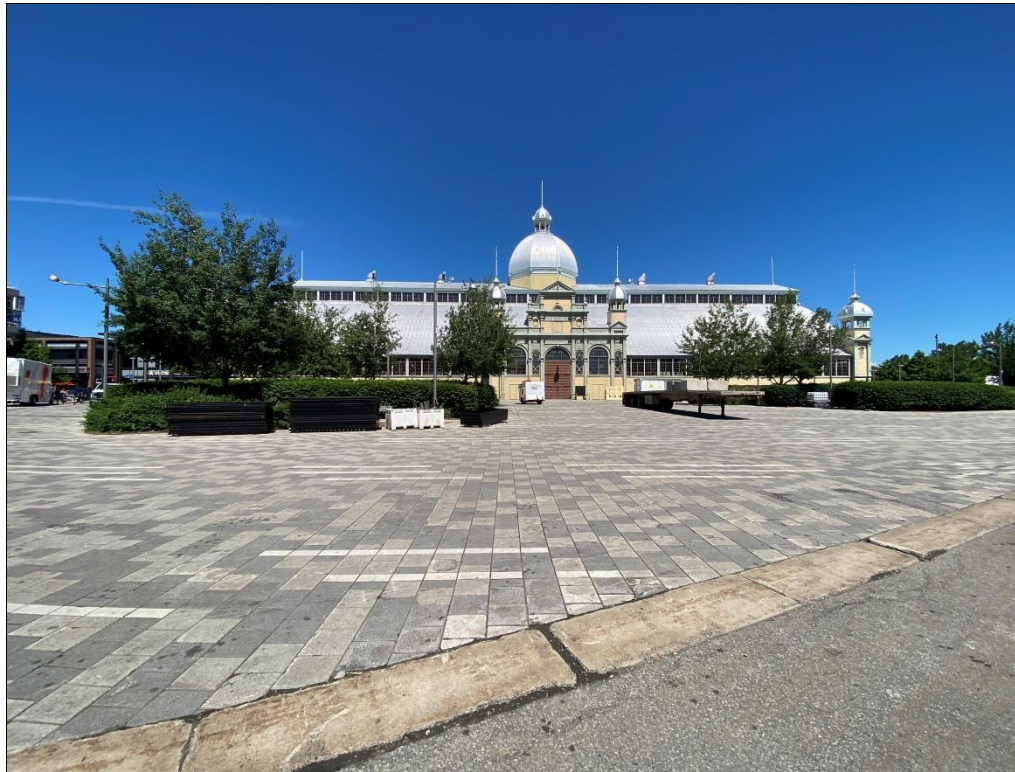
Photo 5: General view of the south elevation of the Great Porch area. Date: 06/28/24 Direction: Northwest
