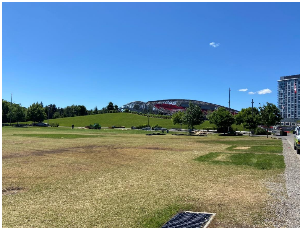
Photo 8: General view of the eastern elevation of the East Berm. Date: 06/28/24 Direction: Southwest
