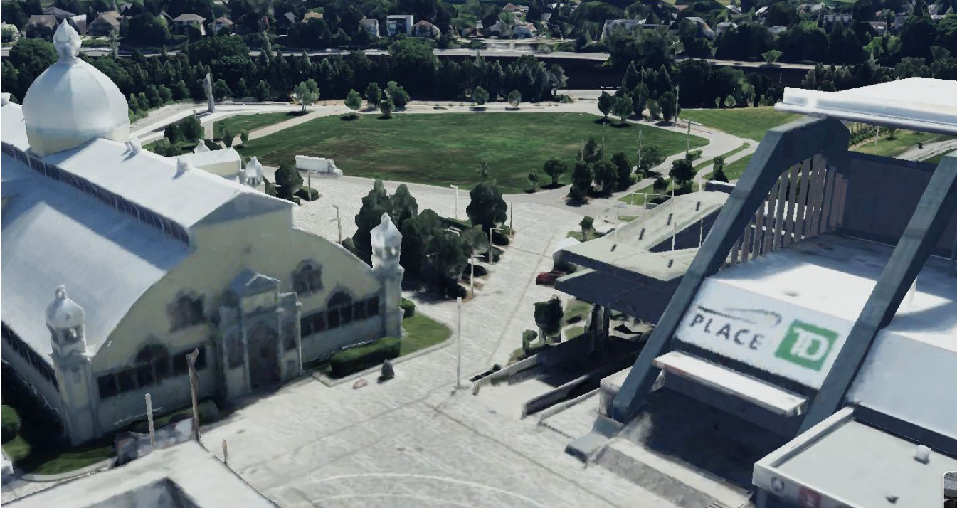
Figure 6. Existing condition looking south-east.
