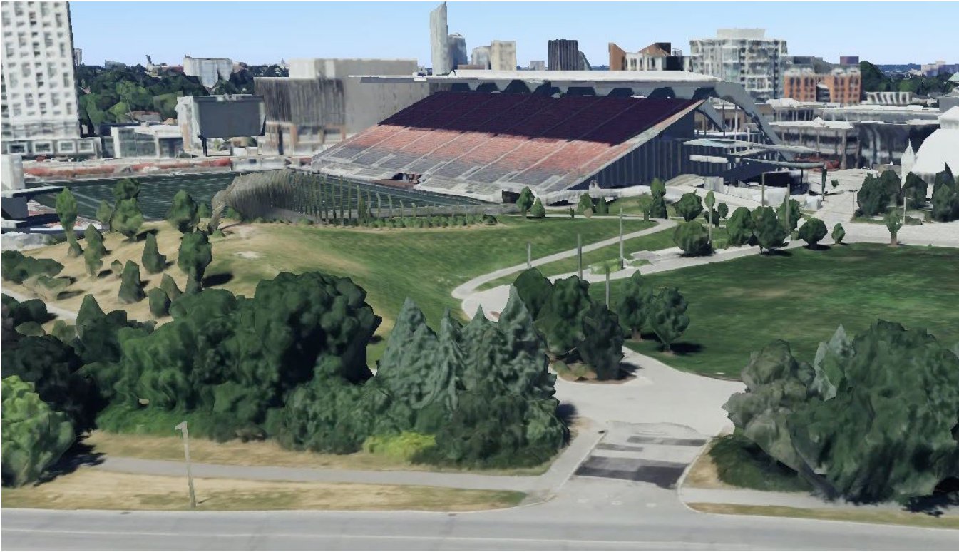
Figure 5. Existing Condition looking north-west.
