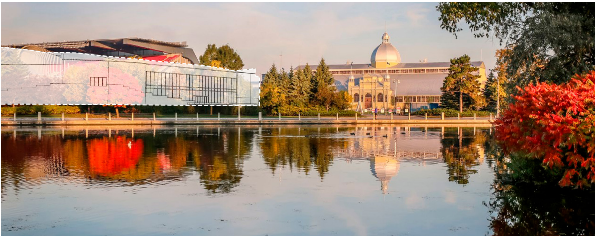
Dynamic view along the Rideau Canal, proposed condition (Rideau Canal Cultural Landscape Study, Matrix Heritage, 2024 DRAFT, annotated by ERA).
