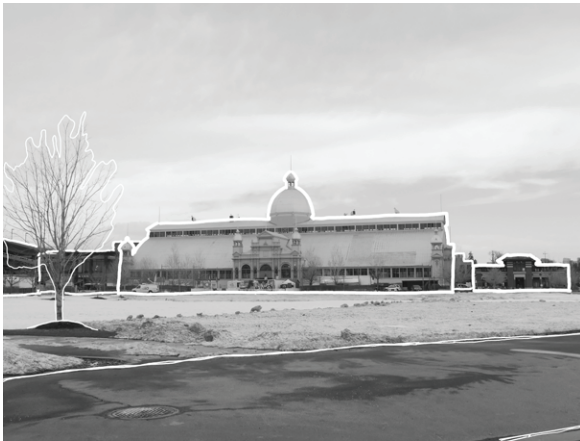
Existing condition of Viewpoint A.
