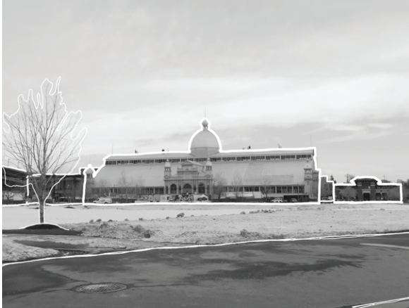
Existing condition of Viewpoint A.
