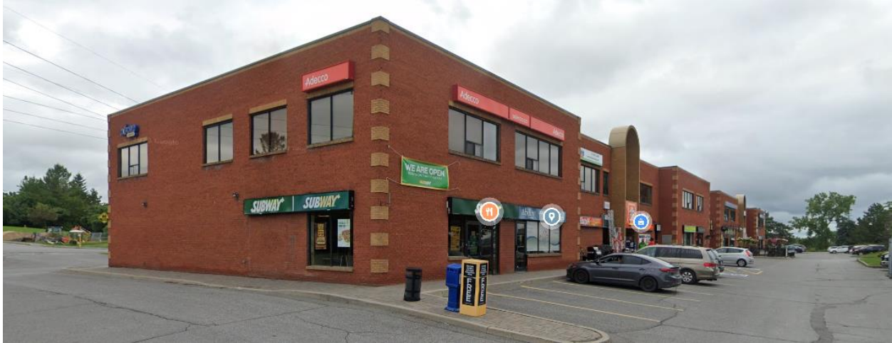
Figure 22: Existing Commercial Plaza, 329 March Road.
