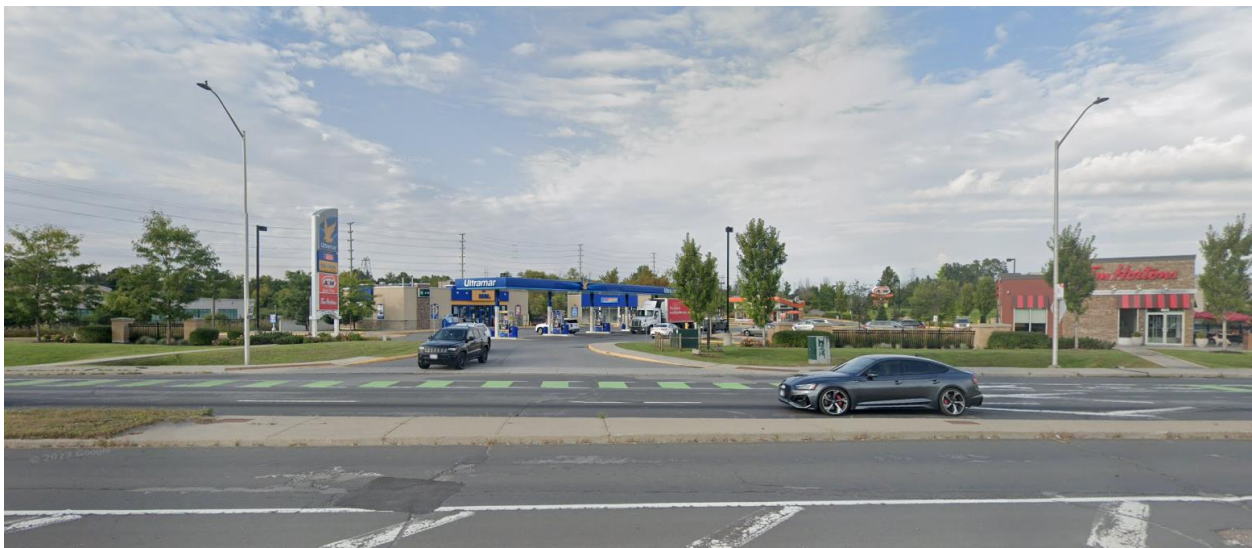
Figure 23: Existing Commercial Plaza, 401 March Road.
