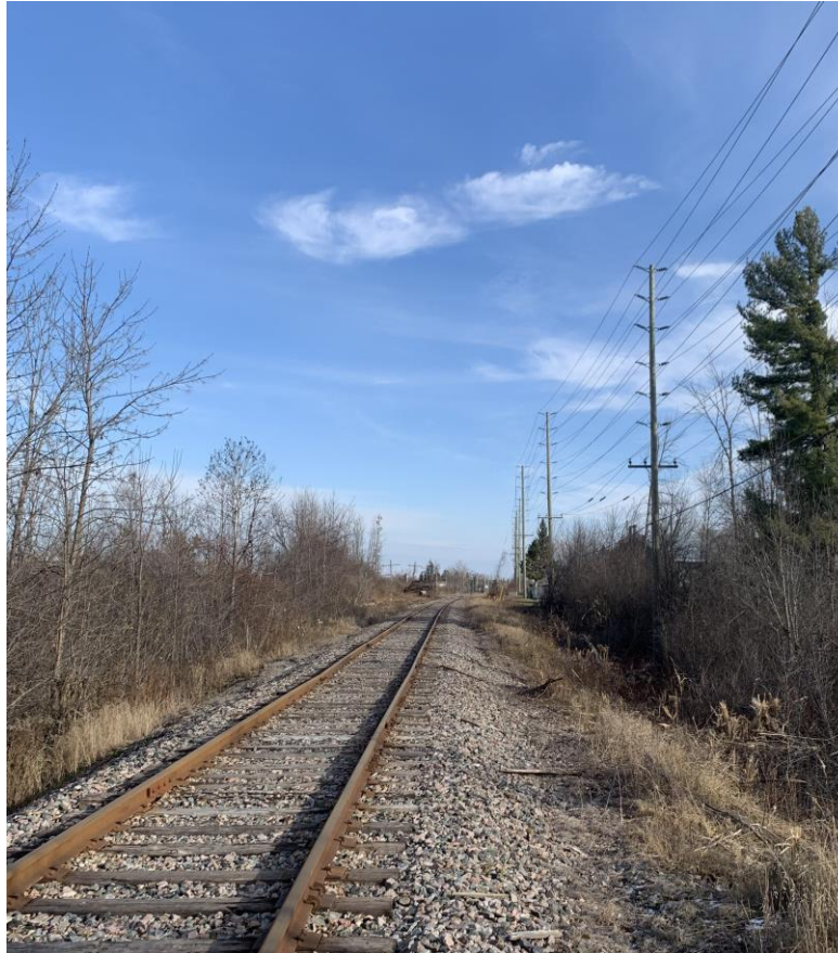
Figure 28: Beachburg/Renfrew Railway Corridor, looking East
