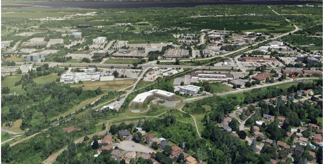
Figure 38: Aerial Image of the proposed development, facing North-East.
