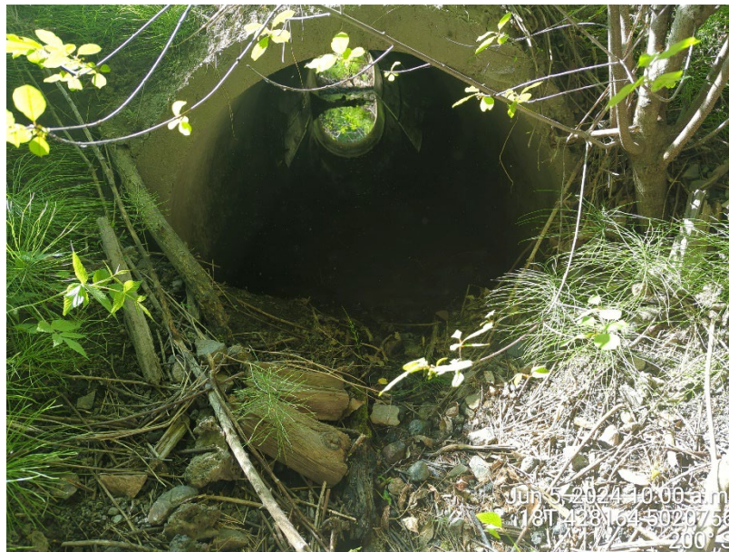
Photo 2: Culvert under the Railroad (June 5, 2024)
