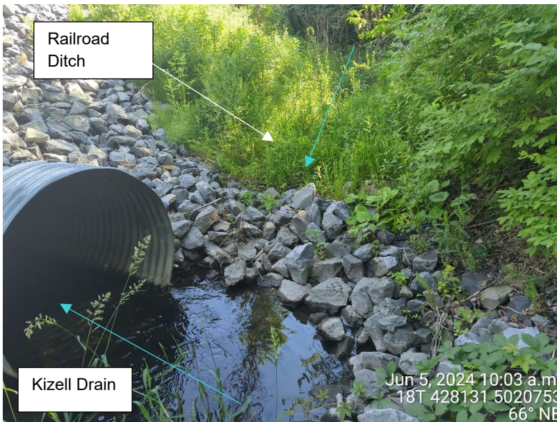
Photo 4: Rip rap at Kizell Drain creating a barrier at the downstream end of the ditch (June 5, 2024)
