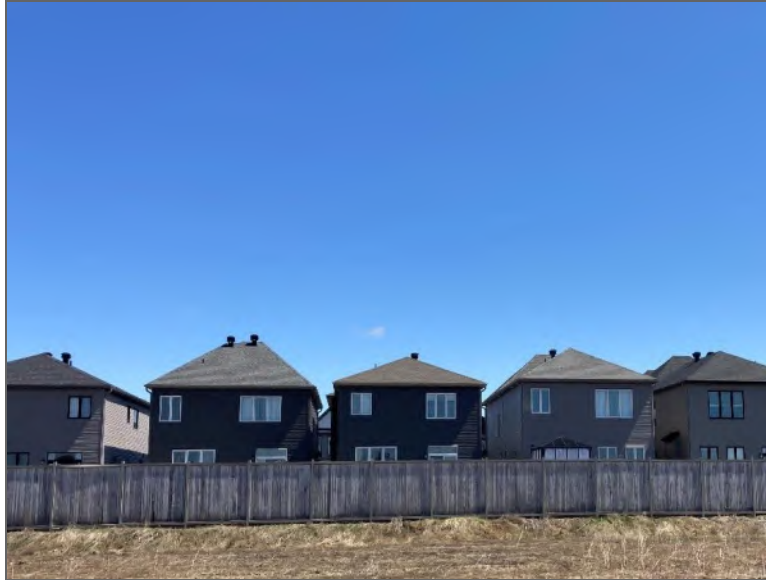
Photo 7 – Properties located east of the Phase One Property.
