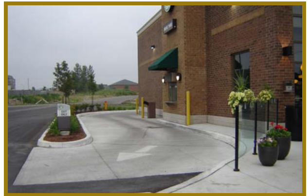
An example of a drive-through aisle distinguished through use of alternate surfacing material.
