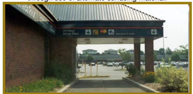
This drive-through facility provides an attractive portico with a soft landscaped edge to delineate the drive-through aisle.
