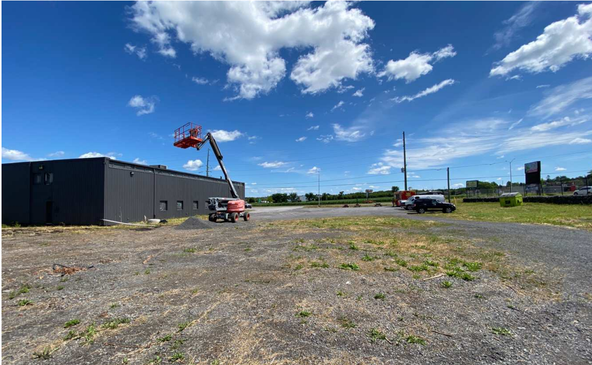
Figure 9: View of the site from the rear of the property. The building (left in the photo) is located on the subject property.
