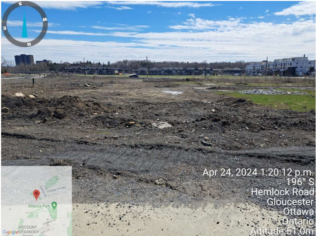
Standing at northside of Street No.1 and looking towards south of Block 5 : No indications of existing slope greater or equal to 2 m in height or any settlement.
