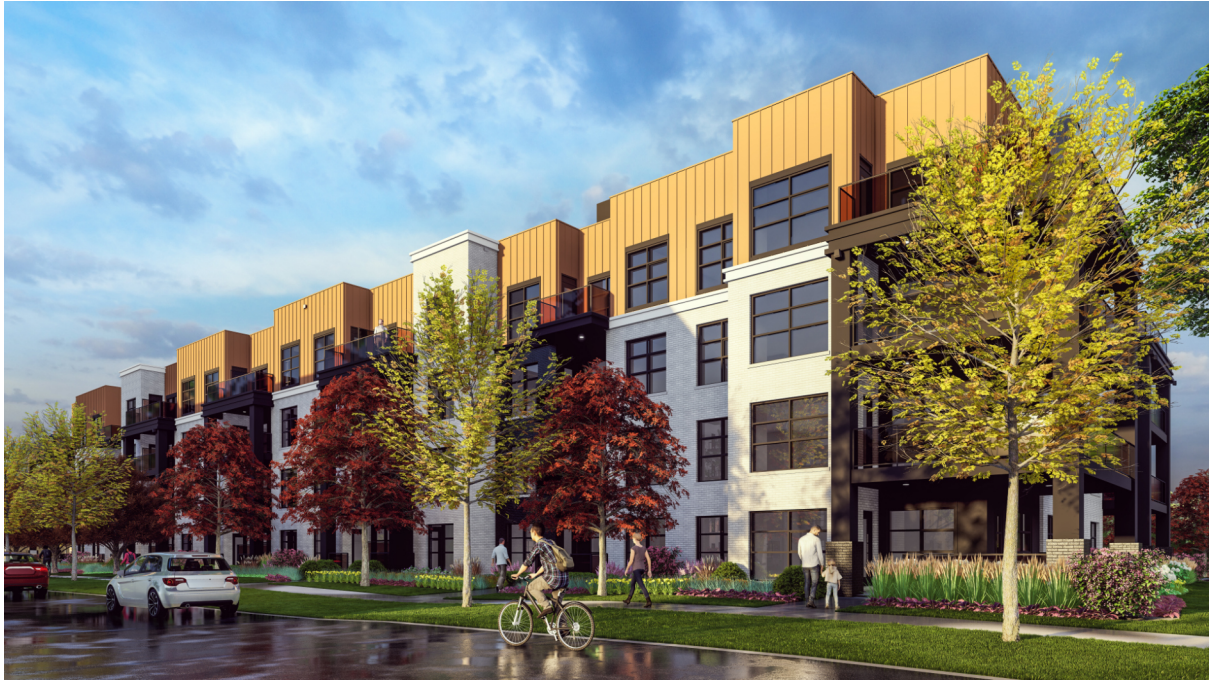
Figure 13.2 – Looking southwest towards the site along Oshedinaa Street (March 2024).
