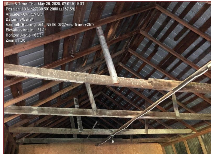
Site Photograph 4 – Inside Roof of Barn Structure
