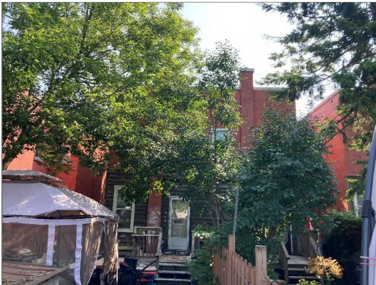
Photo 4 – Site Building B (west elevation).
