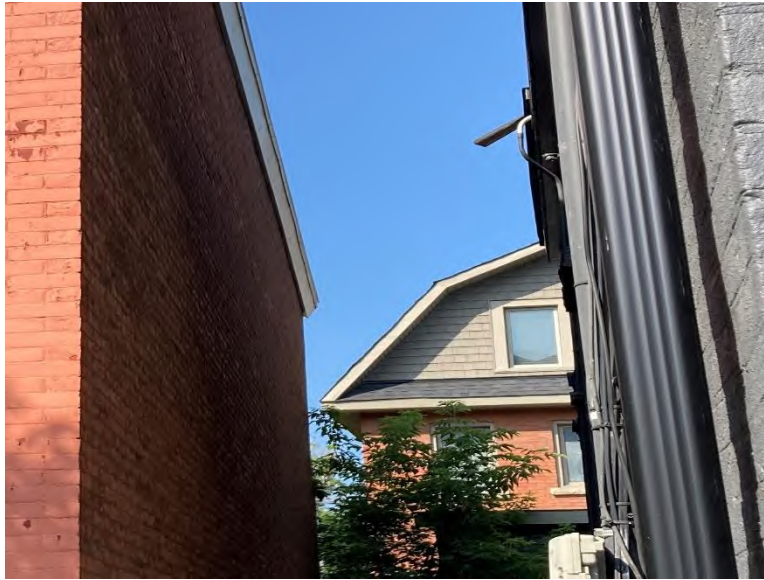
Photo 1 – Site Building A (north elevation).
