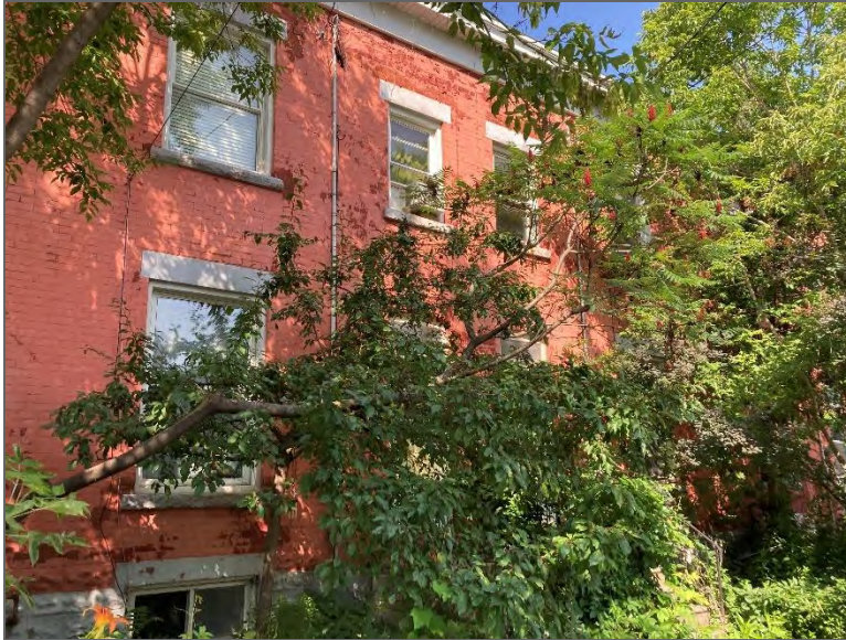
Photo 3 – Site Building A (east elevation).
