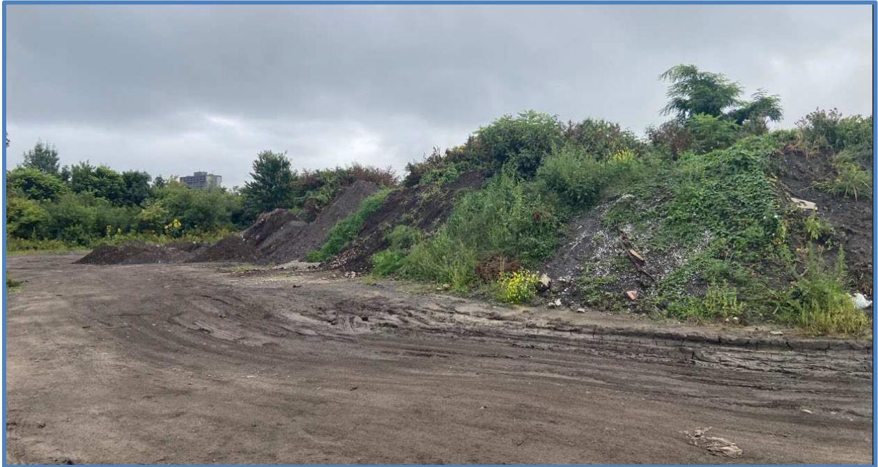
Figure 9: Unconsolidated Fill Piles.
