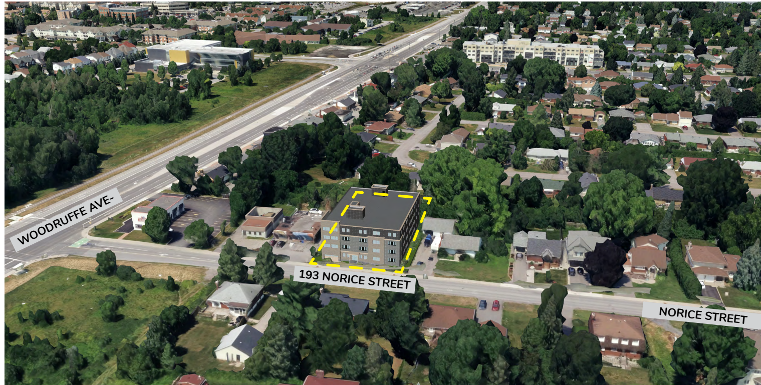
1 - AERIAL VIEW NORTH WEST ALONG NORICE STREET
